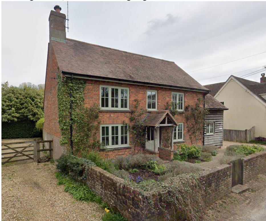
Fig 7 – View of the Glencoirn house street elevation.
