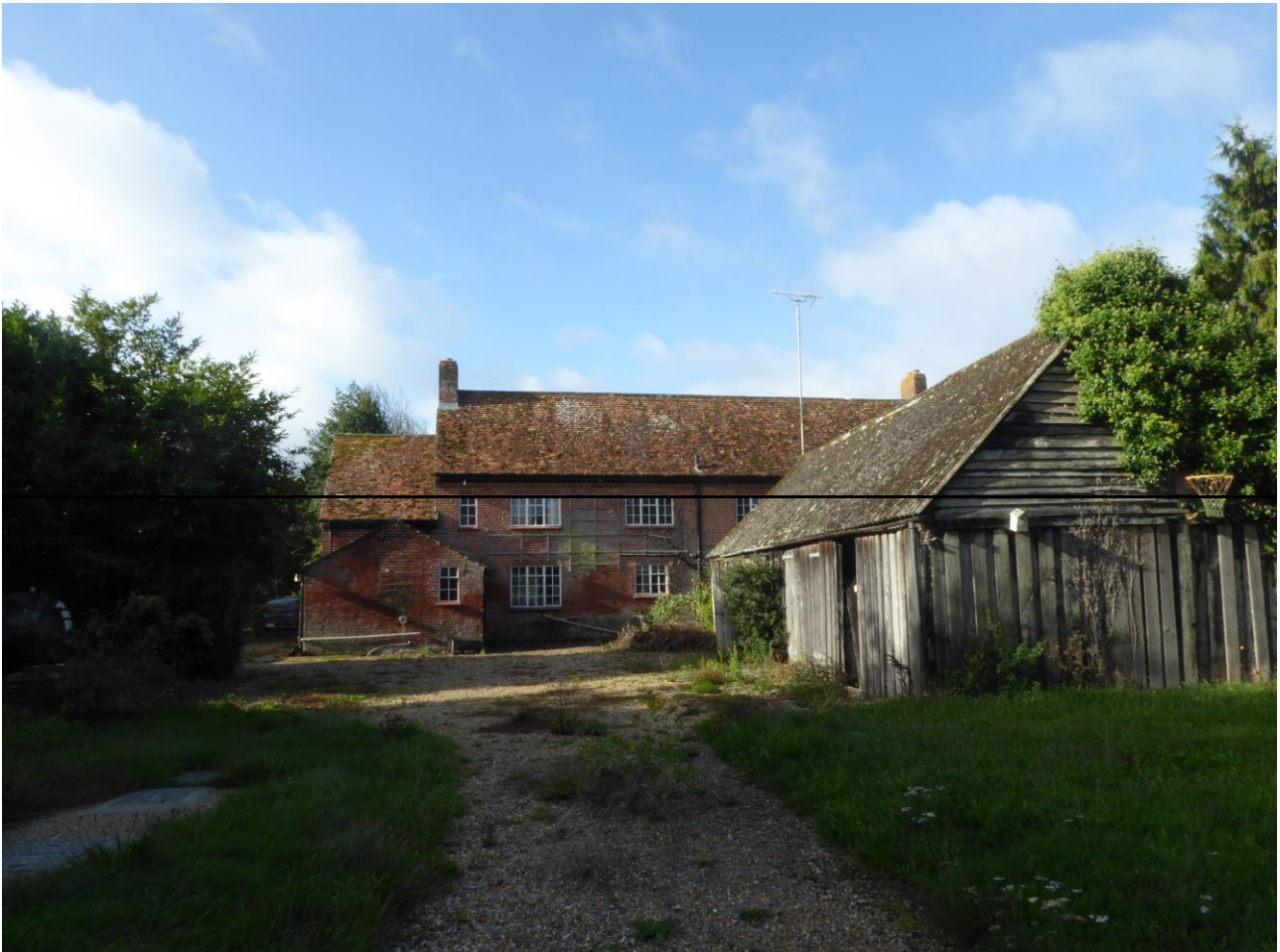
Fig 1 – View of rear elevation and outbuilding and parking area looking south west.
