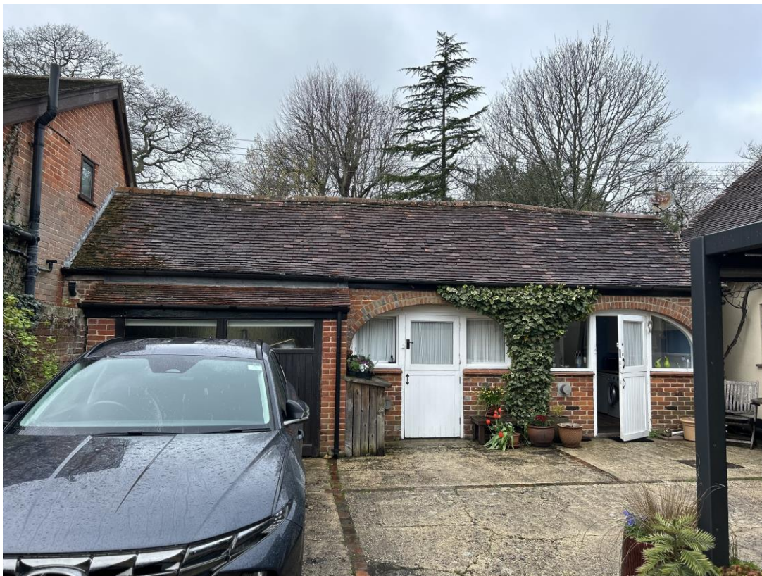
Photo of site from east, with gap between the brick and rendered buildings
