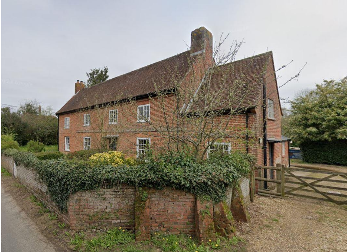
Fig 8 – View of the house southwest elevation from the driveway entrance.
