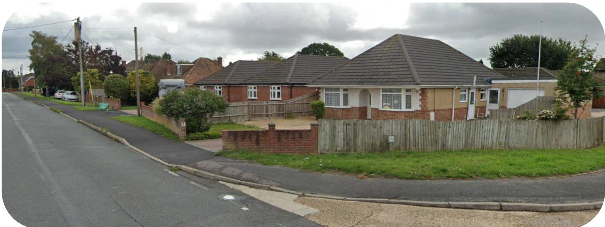
View of bungalows on Holbury Drive just north of application site
