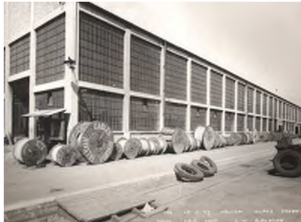
Figure 5. 1937 photograph showing the rolls of telecommunications cable outside a warehouse.
