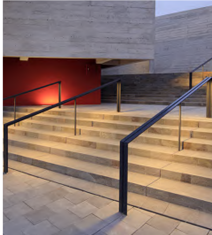
Integral lighting under handrails
