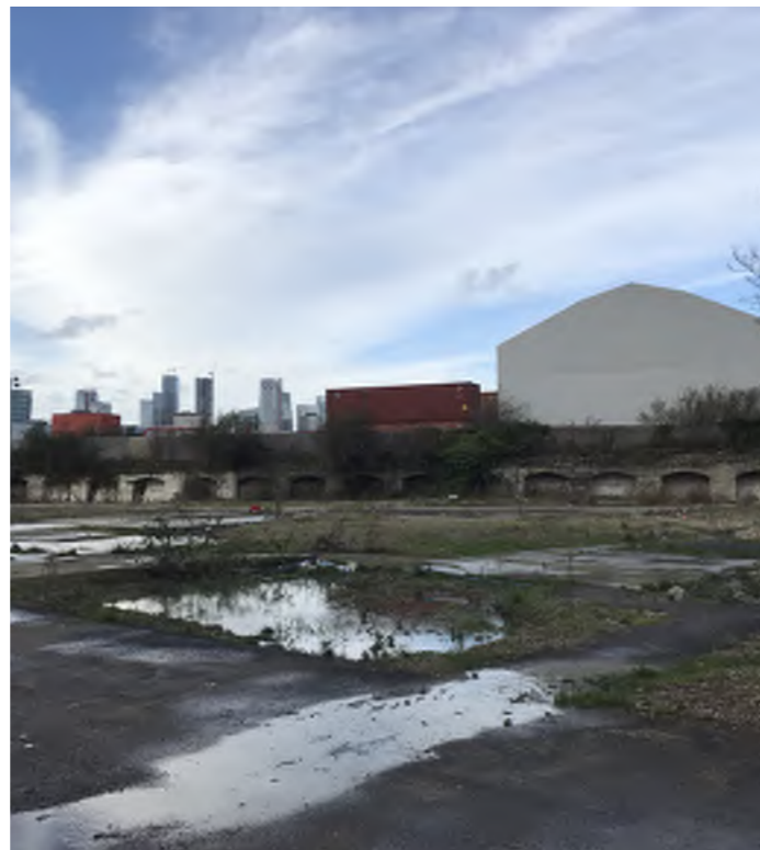
Figure 13. View of the existing retaining wall on Morden Wharf Boundary
