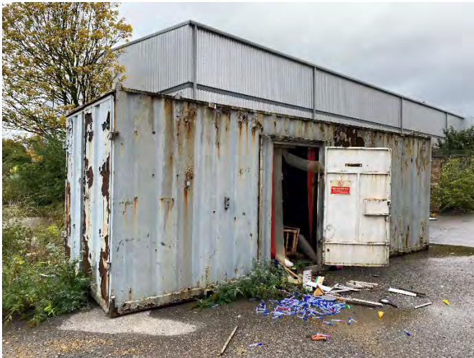
Photograph 2: Building on site
