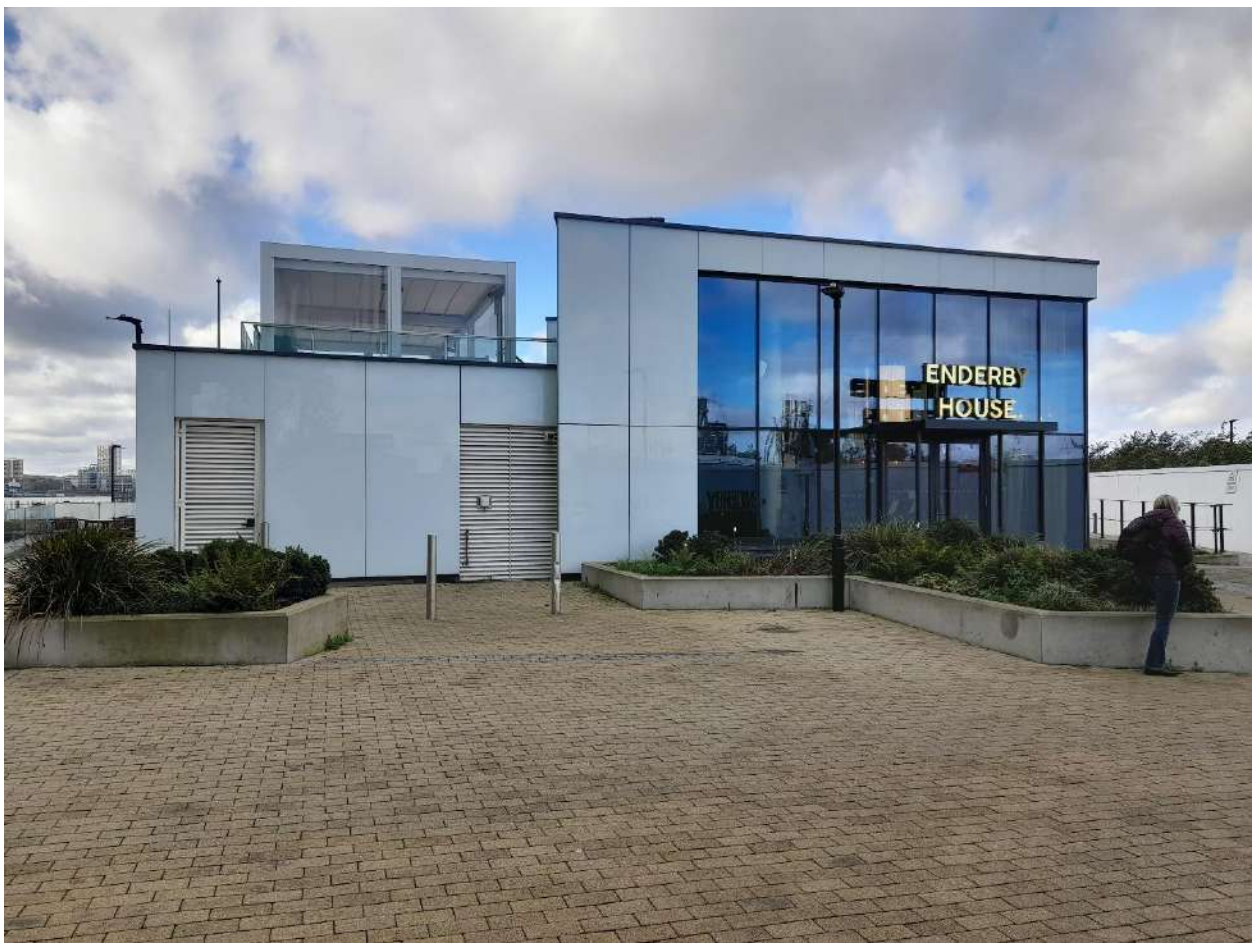
Plate 5: Enderby House. Looking to the west from Telegraph Avenue.
