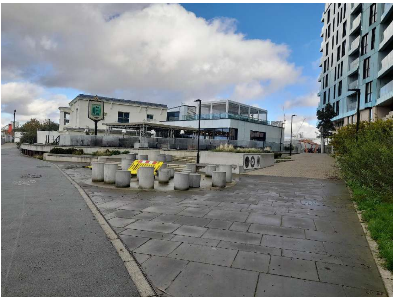
Plate 6: Enderby House. Looking to the north from the Thames Path.
