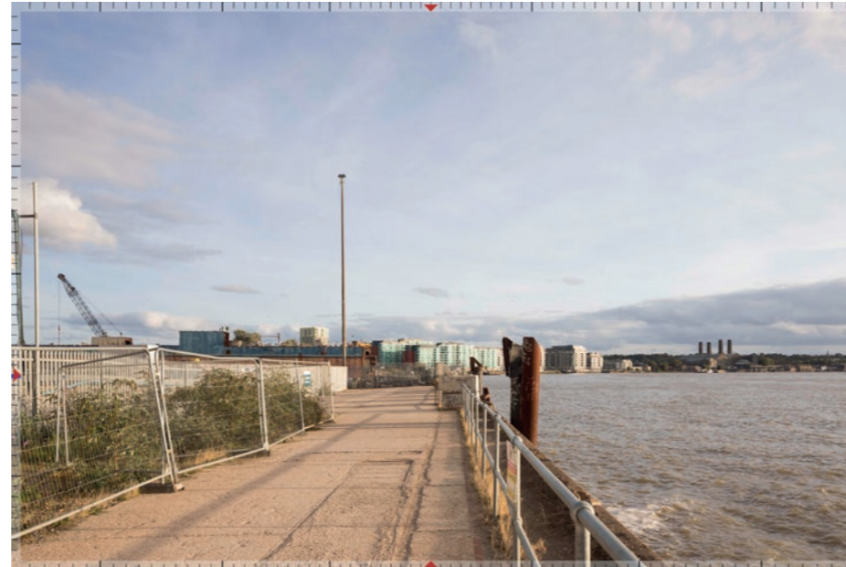
Figure 3.33 View 23: Riverside Walkway (Existing). Source: Miller Hare
