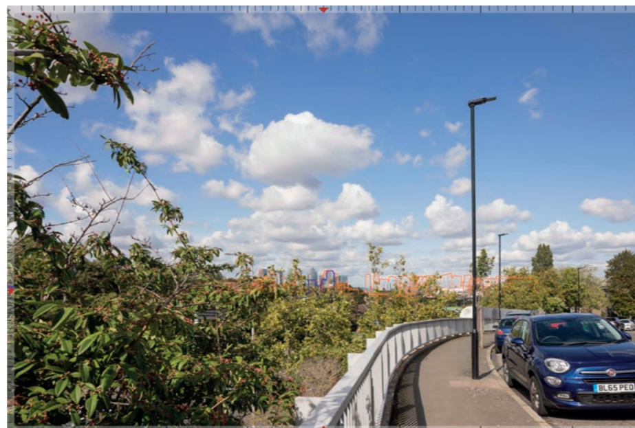
Figure 5.39 View 16 Charlton Road Bridge over the A102 (Cumulative). Source: Miller Hare
