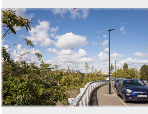
Charlton Road Bridge over the A102 - Existing 7027_2201 version 231016
