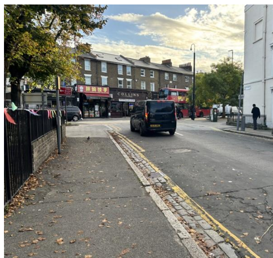
4. Christchurch Way (north of Trafalgar Road)
