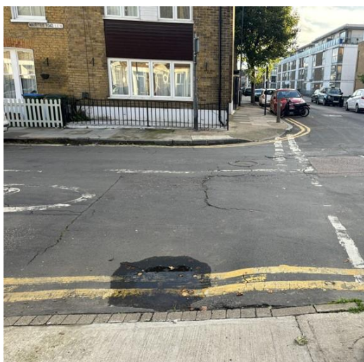
1. Christchurch Way (at Mauritius Road)
