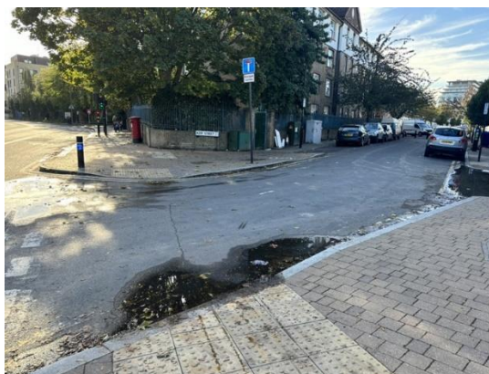
3. Blackwall Lane (at Azof Street)
