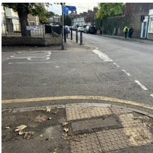
3. Christchurch Way (at Pelton Road)
