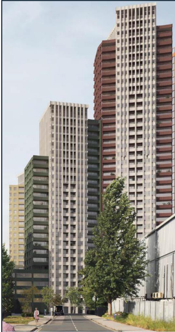
Figure 5.8: Illustrative Image Looking West at the Development from Telcon Way (Source: DAS)
