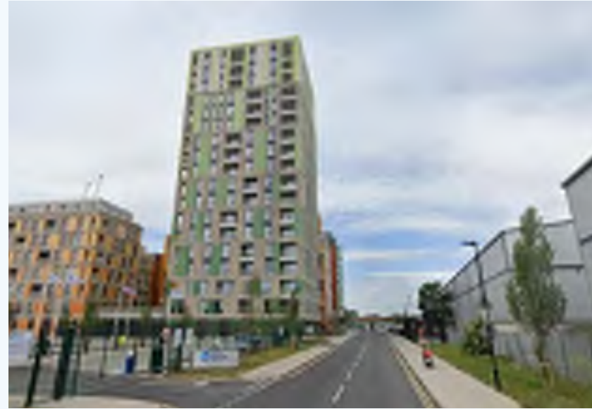
TELEGRAPH WORKS (19S) ADJACENT TO LOW RISE INDUSTRIAL BUILDINGS
