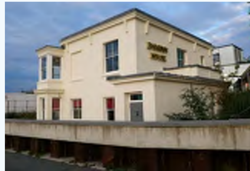
ENDERBY HOUSE - LISTED BUILDING
