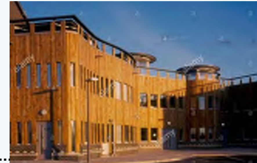
MILLIENNIUM PRIMARY SCHOOL & ST MARY MAGDALENE C OF E SCHOOL PENINSULA SITE - 20 MIN WALK
