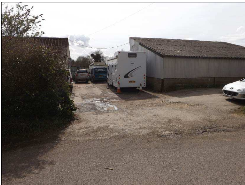
Plate 3: General view of the buildings on the site looking south.
