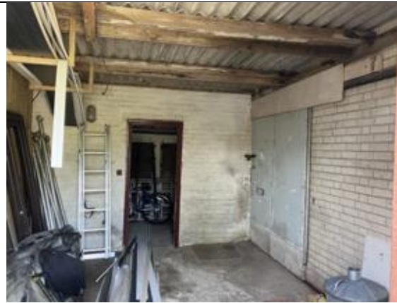
Photograph 8. Inside the workshop with brick build and no lining
