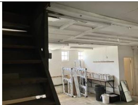
Photograph 10. Inside the workshop
