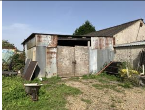
Photograph 12. A corrugated store with overlapping corrugated metal sheets and chrysotile roof.
