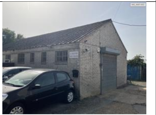
Photograph 16. Brick build garage, with metal shutter door.
