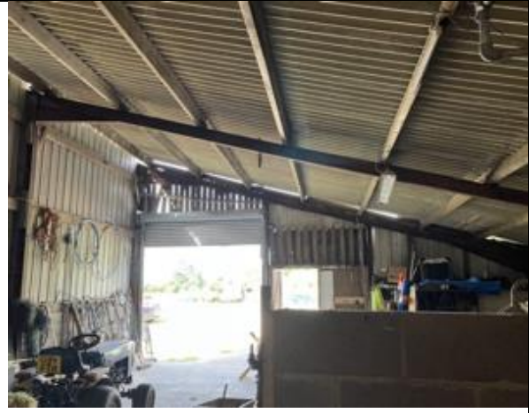
Photograph 14. Internal view of the agricultural barn
