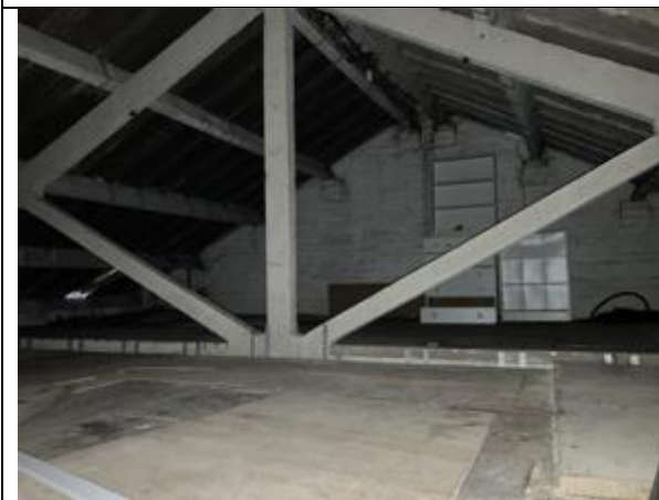
Photograph 9. Internal space above the workshop.
