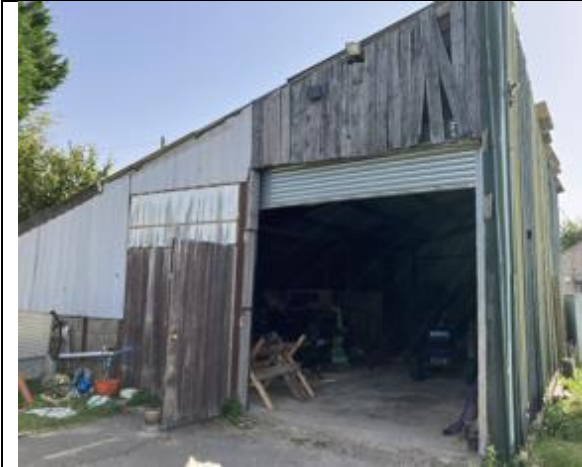
Photograph 13. Agricultural barn with breeze block plinth and steel frame
