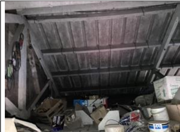
Photograph 7. Internal roof void above the garage
