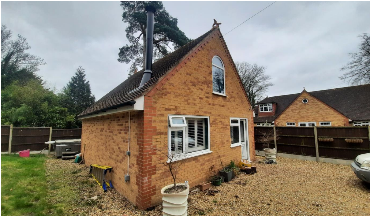
View of northwestern corner to annex.
