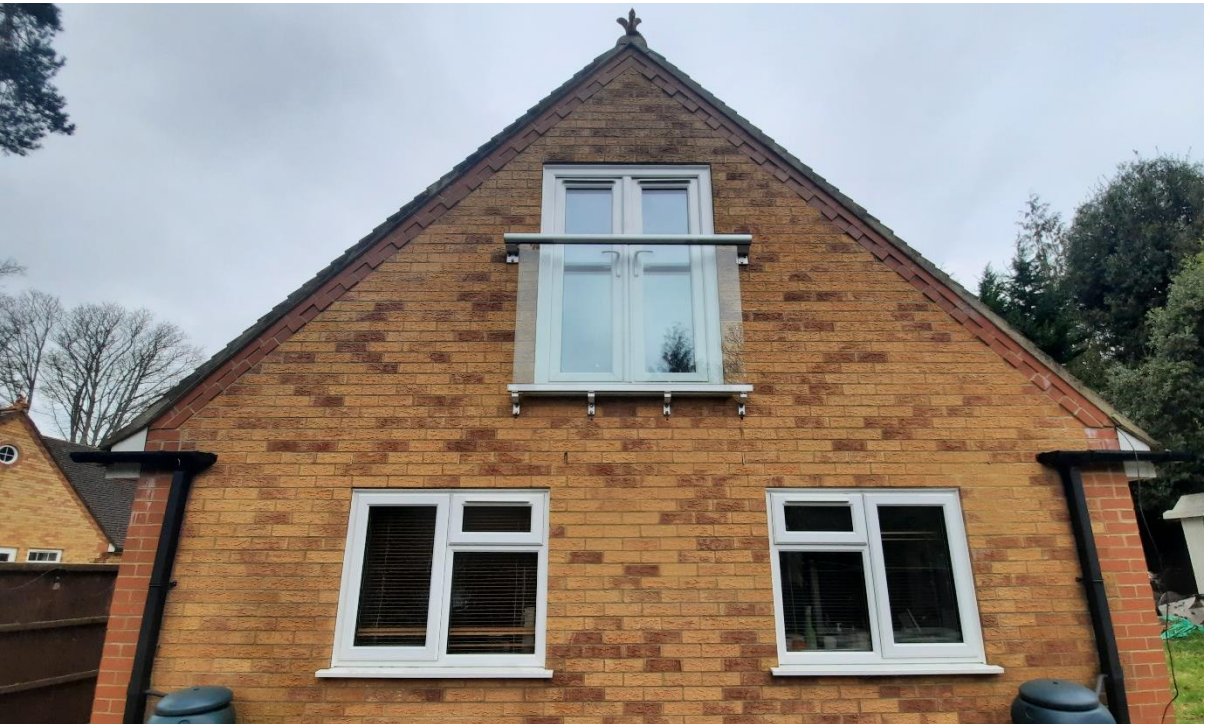
View of annex rear elevation to the east.
