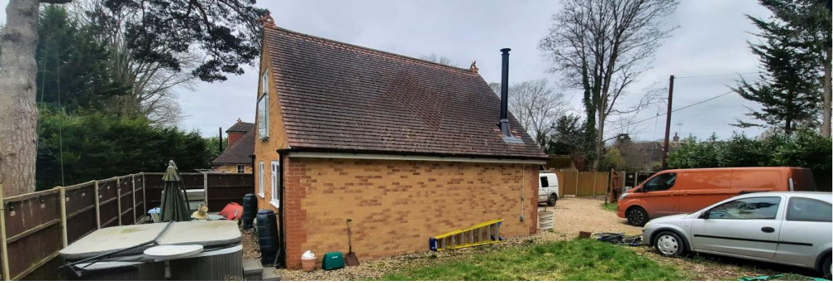
View of annex side elevation to the North.
