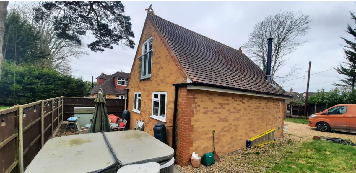
View of northeastern corner to annex.
