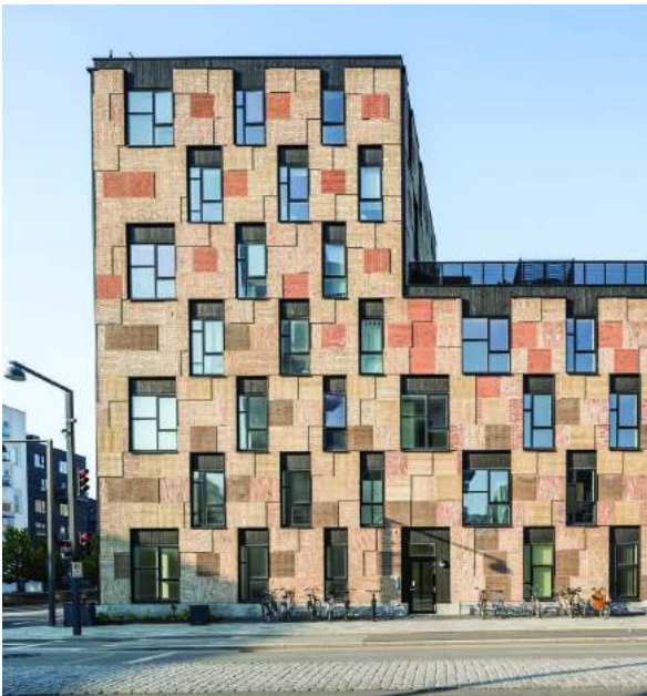
Fig 2. Example of Brick reuse - Brick Facade Panel - Source: Lendanger, Resource Rows Brick mounted on-cement board panel. This could be an option for re-using the existing brick wall if disaggregation to brick is not effective.
