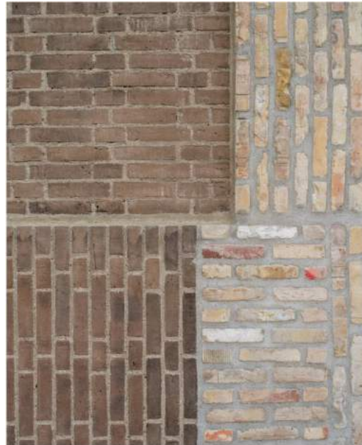
Fig 2. Example of Brick reuse - Brick Facade Panel - Source: Lendanger, Resource Rows Brick mounted on-cement board panel. This could be an option for re-using the existing brick wall if disaggregation to brick is not effective.
