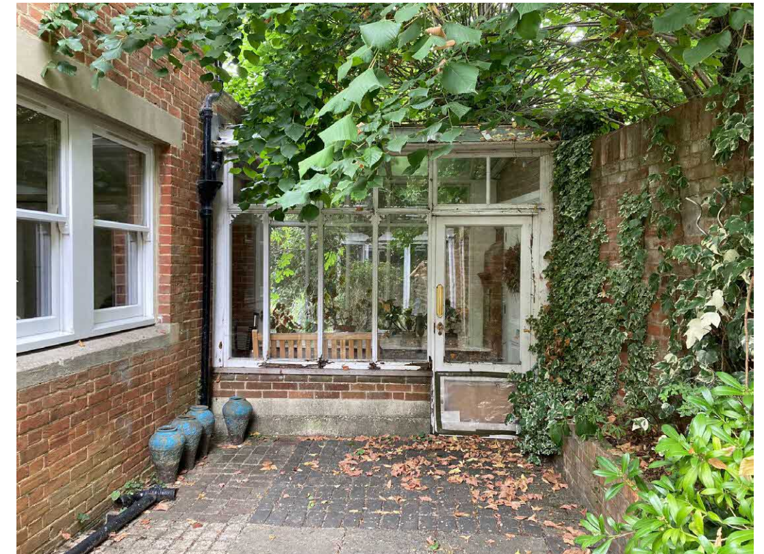
Figure 9. Existing courtyard access. South elevation.
