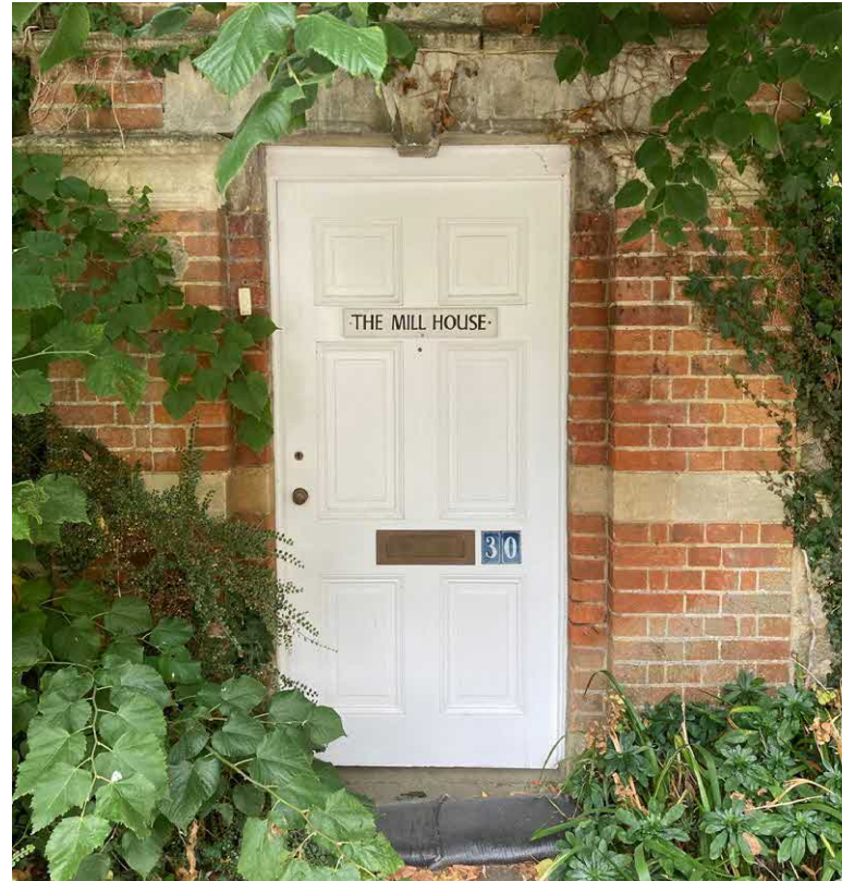
Figure 6. Existing site access. East elevation.
