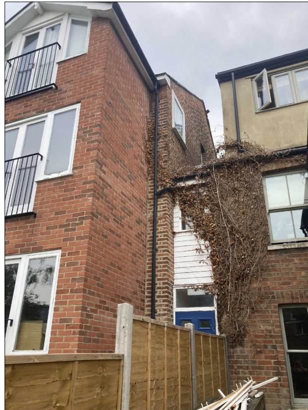
View towards neighbour at no. 72
