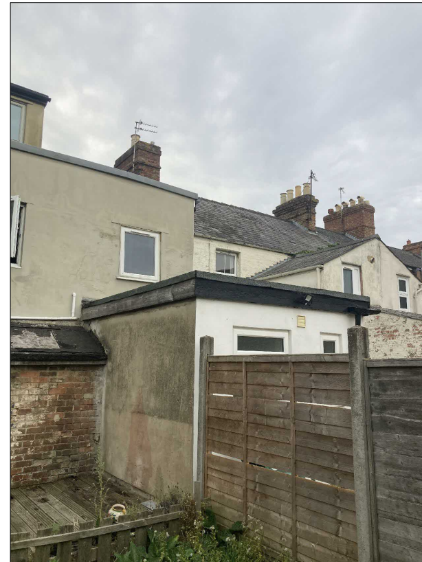
View towards neighbour at no. 70
