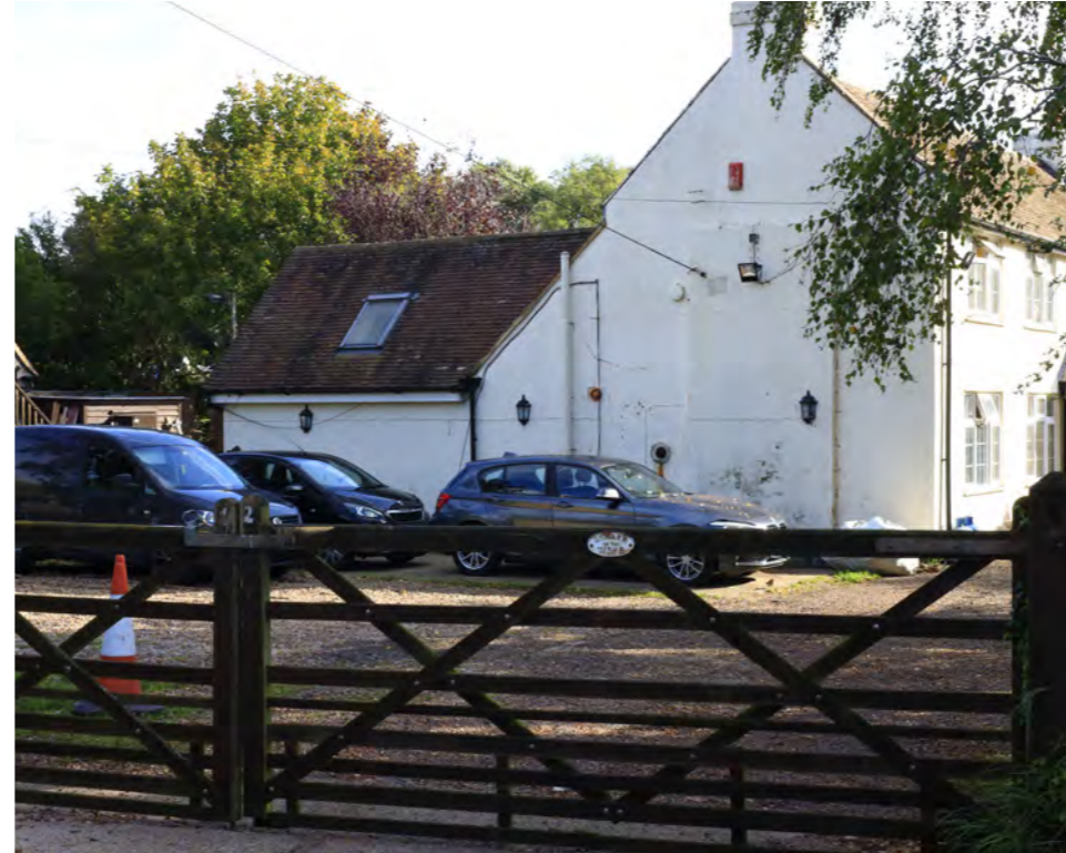
02: Brickfield Cottage [Eastern Edge of Richborough Road]
