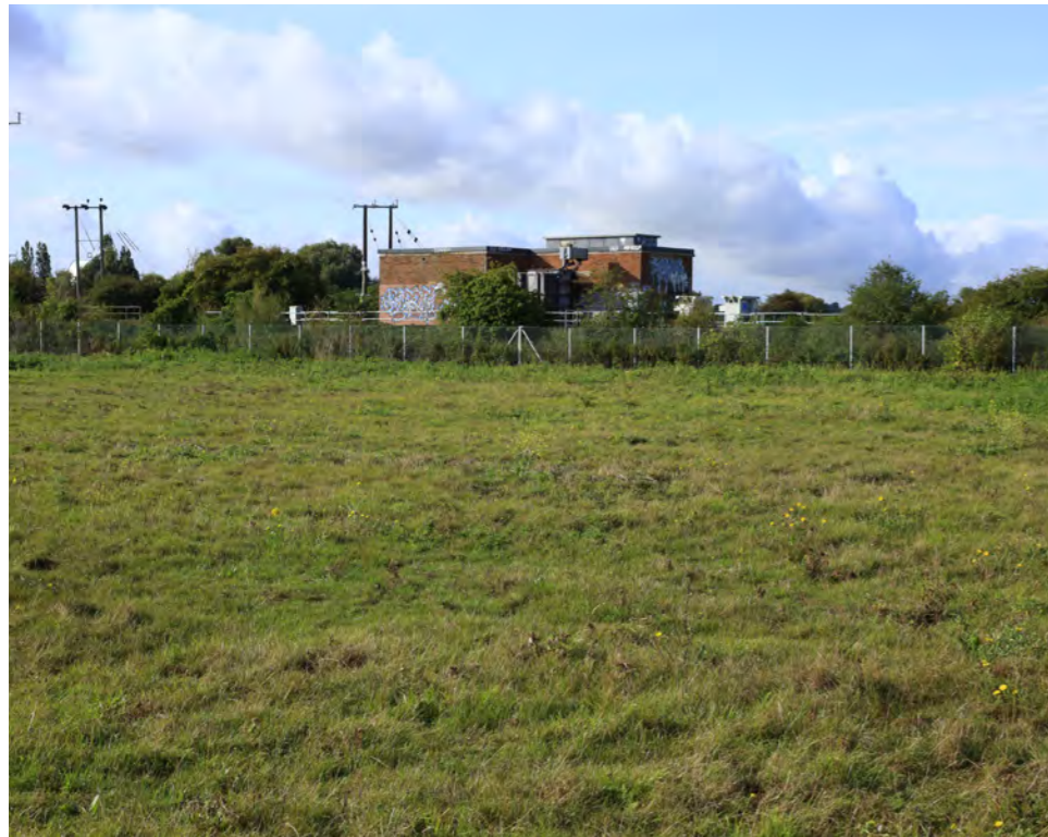
10: Railway Embankment & Associated Buildings
