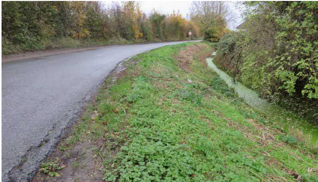
Photo 1: Deep ditch along the west side of Richborough Road
