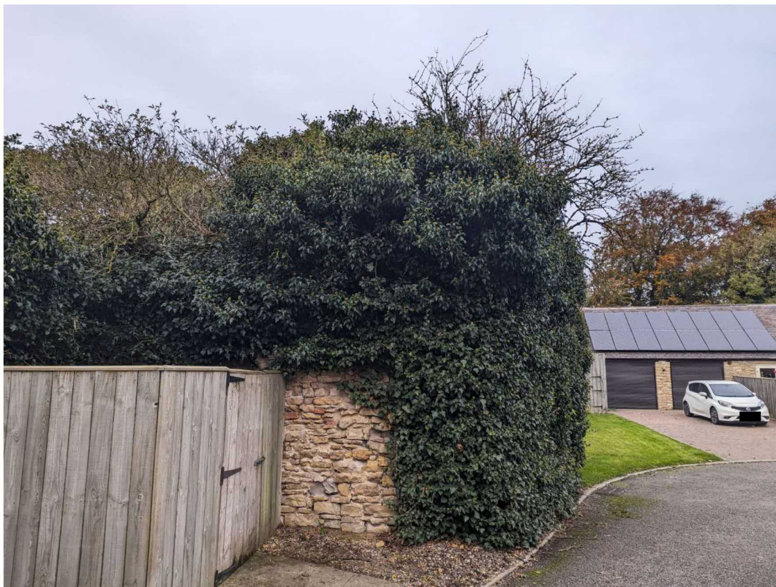
Figure 4 – Vegetation to gable elevation
