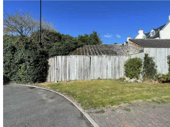
Photo of Rear Elevation
