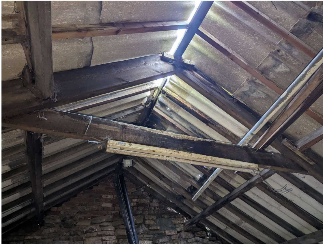
Figure 3 – Existing roof structure
