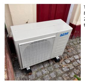
The new external condenser is 654mm high by 855mm wide and a depth of 328mm, it operates at 29dB which for reference is considered to be quieter than a whispered conversation.
