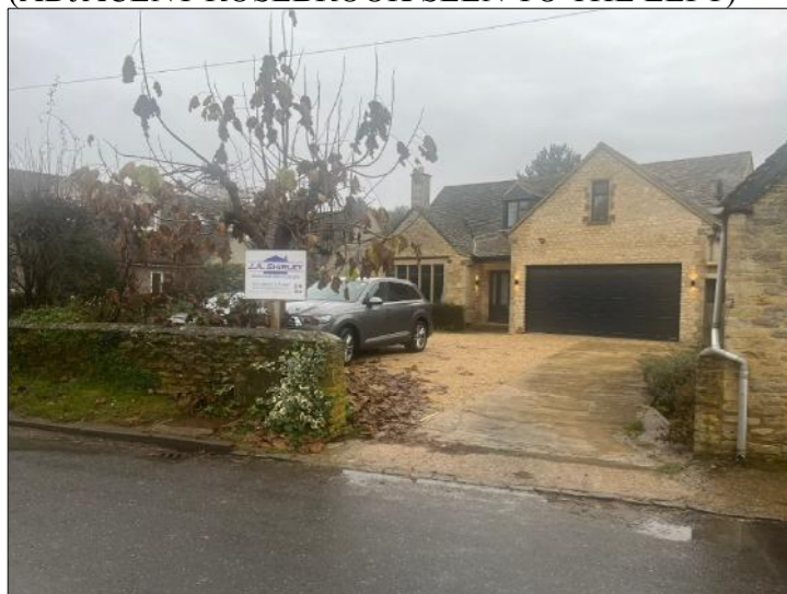
HOUSE FROM THE ROAD (NOTE POOR CONDITION TREE)
