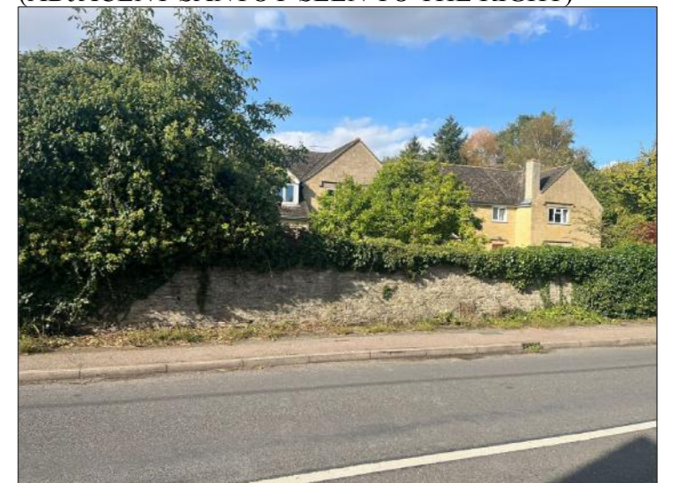
EXISTING WALL OPPOSITE AT CIRCA 1.7m HIGH
