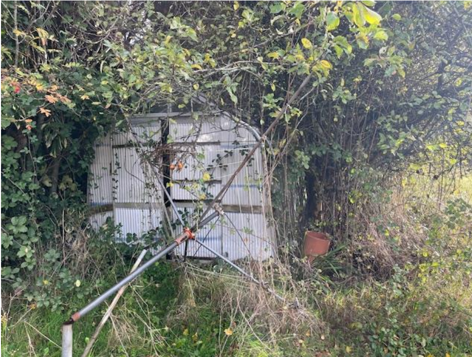
Sheds to be demolished
