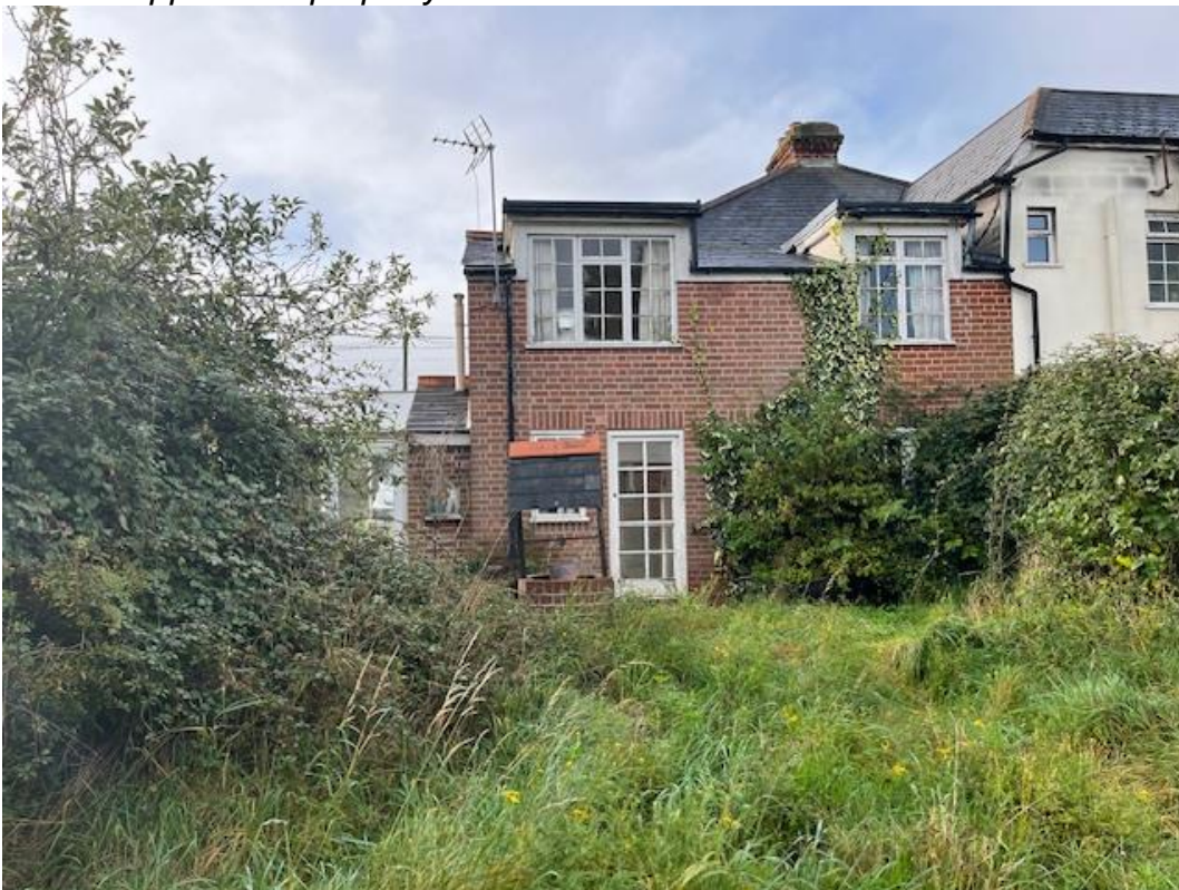
Rear of application property
