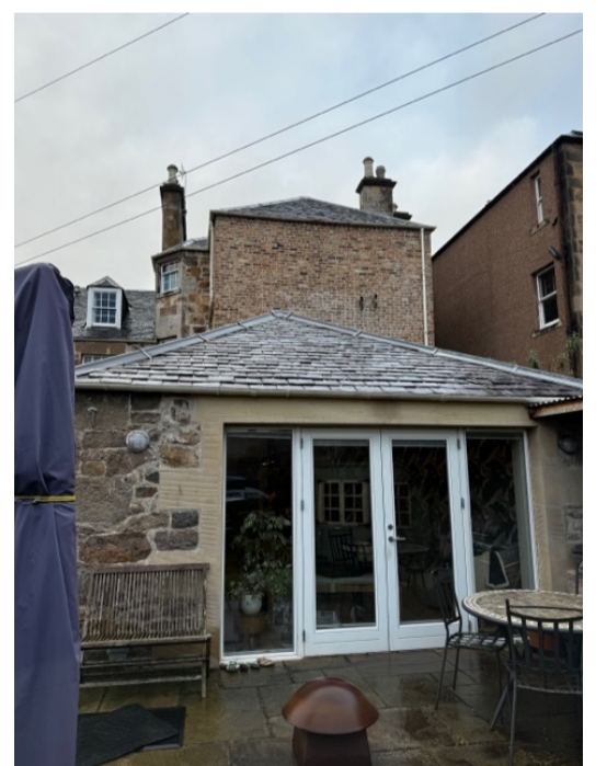
Photo showing existing west elevation
