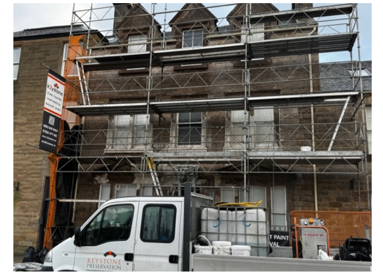
Photo showing existing north elevation (stone cleaning underway)
