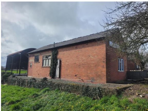
P6: Building B: viewed from the NE, looking SW
