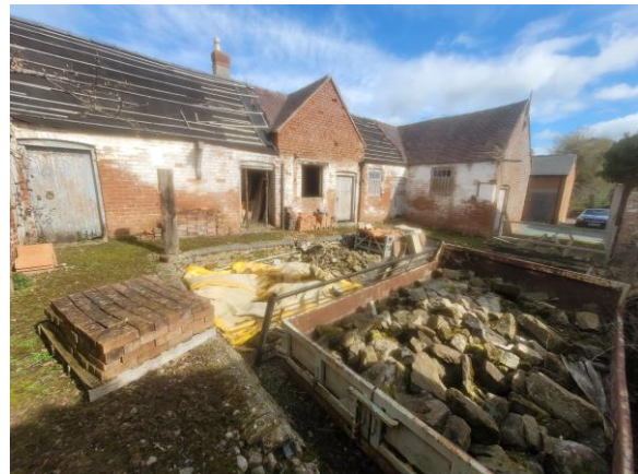
P3: Building A: viewed from the SW, looking NE
