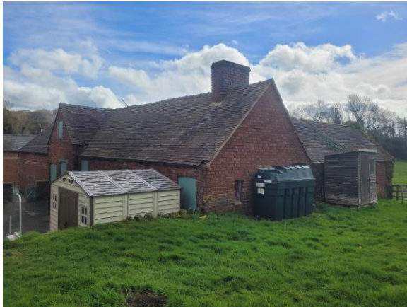
P4: Building A: viewed from the NW, looking ESE
