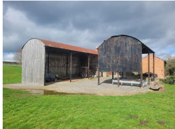
P9: Buildings C + D: viewed from the SE, looking NW
