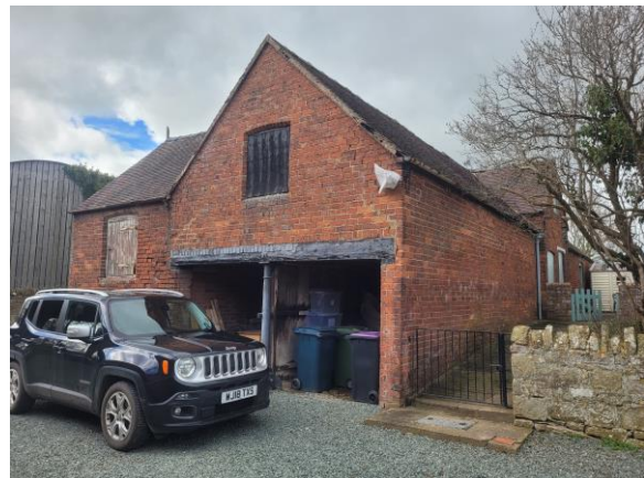
P1: Building A: viewed from the NE, looking WSW
