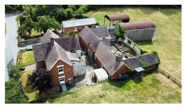
The main farmhouse is a simple brick built cruciform plan vernacular house with plain clay tile roof and steeply pitched gables and sash windows, each light consisting of two panes of sheet glass.
