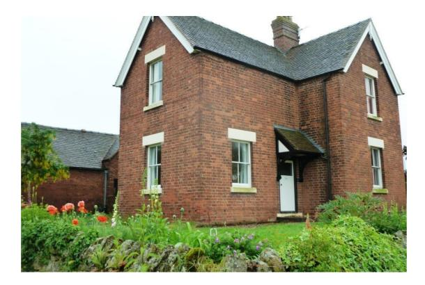
The older windows were constructed in the earlier style of rectangular frame whereas later replacements have projecting horns at the corners to provide greater strength to support the heavy panes of glass.
