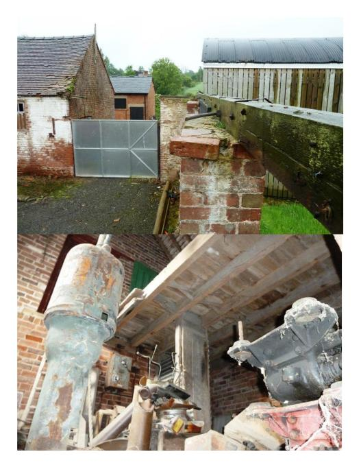
Construction of the buildings utilized the regular shaped bricks of the period probably made in the brickworks at Lebotwood locally. Joinery timber is mostly milled softwood with oak used for key structural items.
