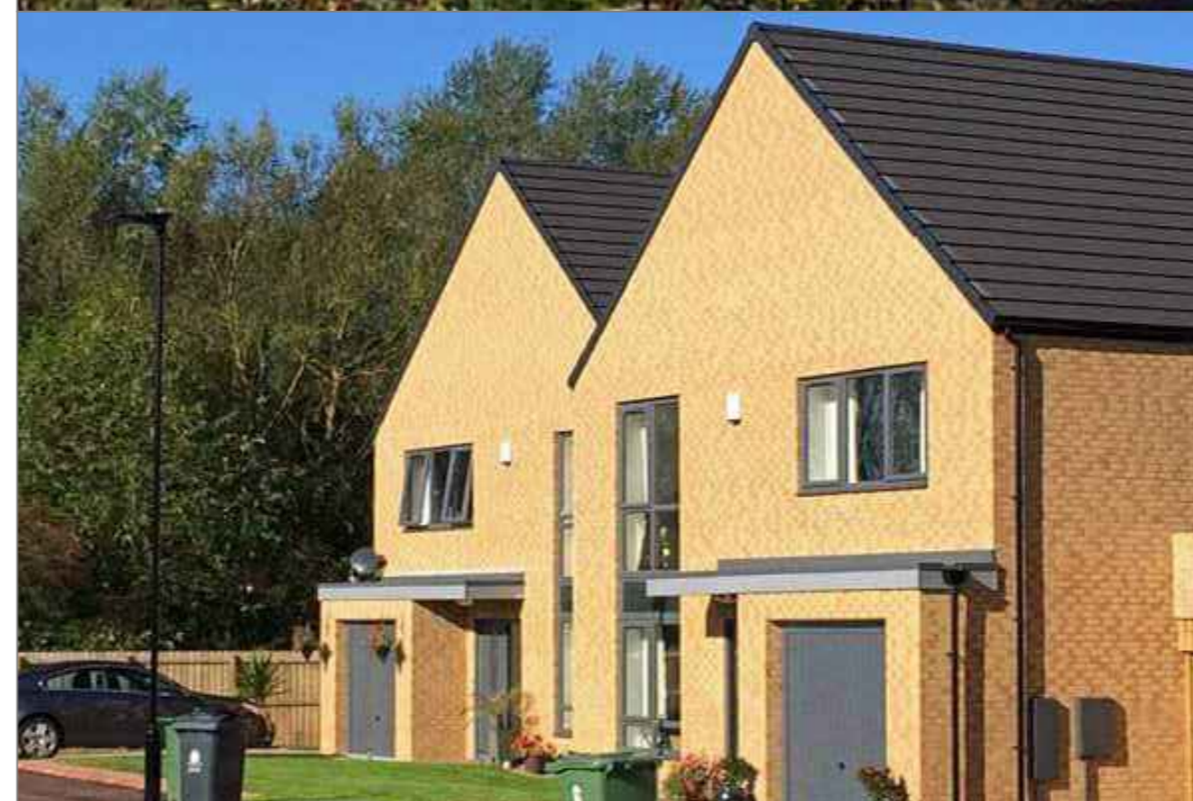
Bricks to be used are Istock Grainger Gold, as shown in the above stock images
