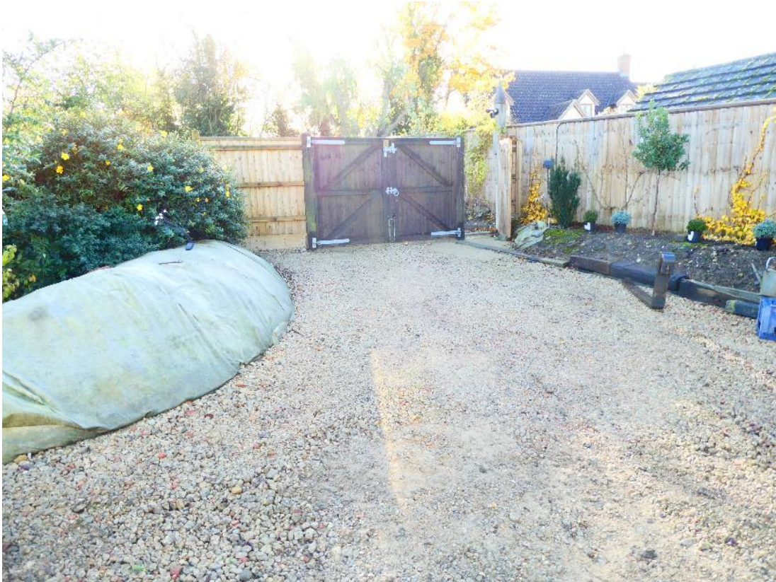
Photo 1 , existing southern compacted gravel hardstanding access to the site, looking southwest.
