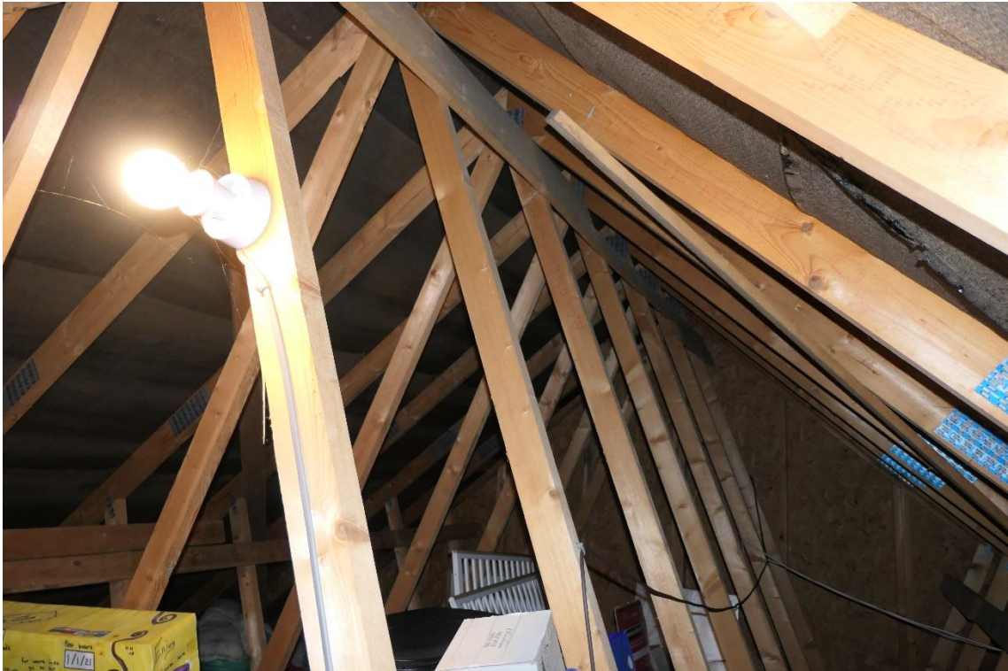
Photo 2 , internal view of building one looking southeast.
