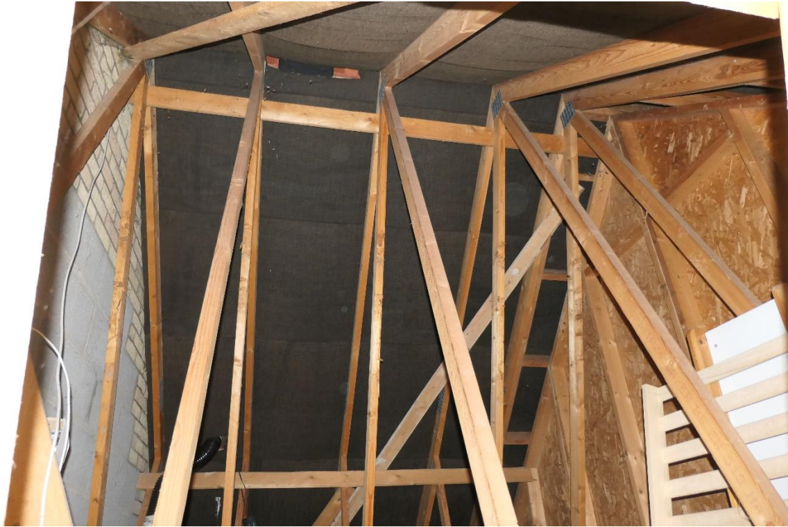
Photo 3 , internal view of building two, looking northeast.
