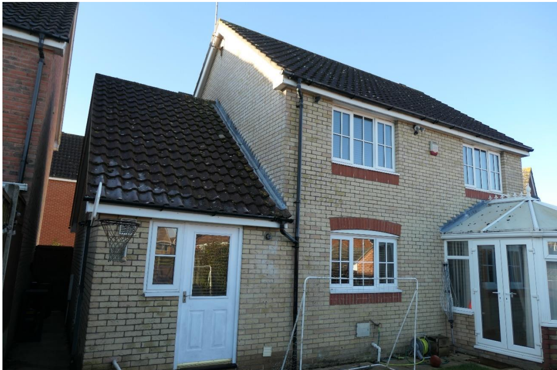
Photo 1 , northeast aspects of building one and two, looking northwest.
