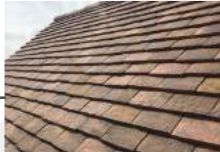
▲ Clay plane tiles to match existing
