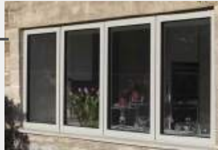
▲ Aluminium composite glazing to all windows - new and existing
