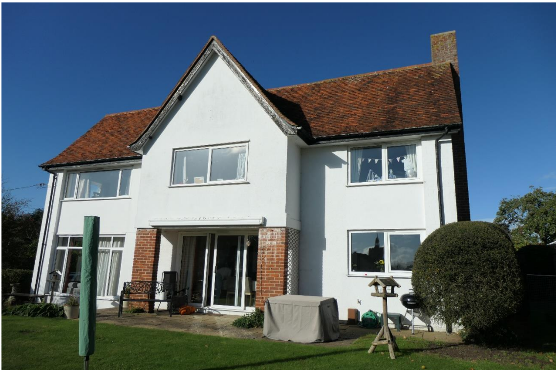
Photo 6 , east aspect of building one, looking west.
