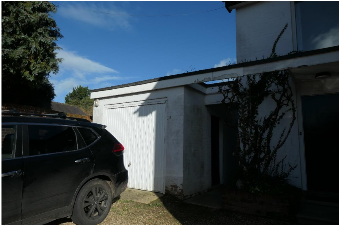
Photo 9 , south and west aspect of building two, looking north.
