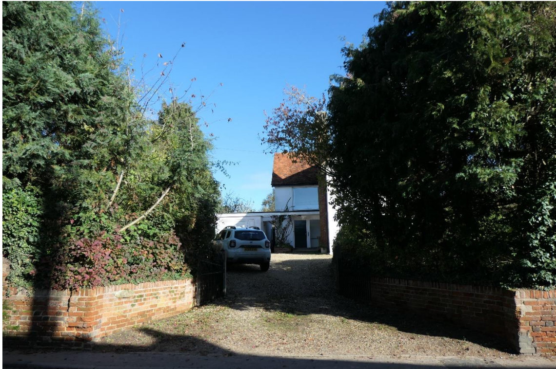
Photo 1 , existing southwestern entrance, looking northeast.
