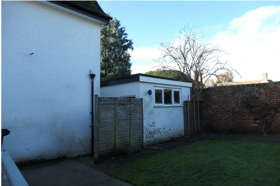
Photo 10 , east and south aspect of building one, looking north.
