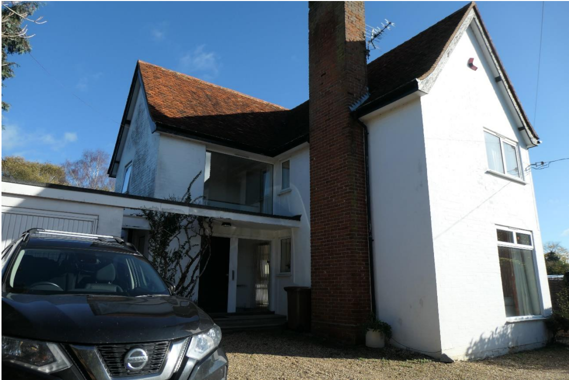
Photo 5 , north and west of building one, looking east.
