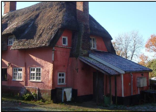
Fig.31 Existing canopy and chimney
