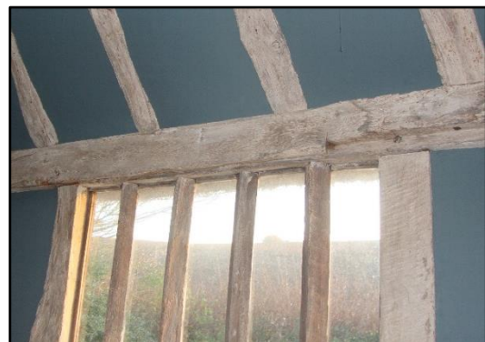
Fig.36 Existing window in chamber
