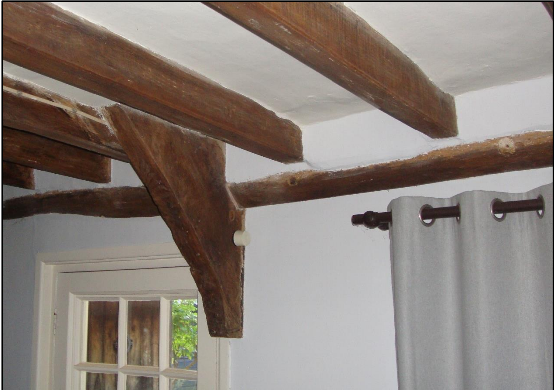
Fig.24 Arch brace of original open truss in hall with later inserted floor
