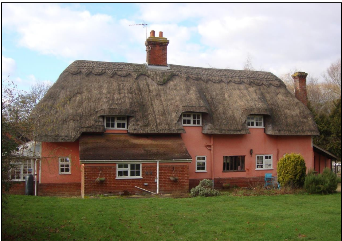
Fig.23 Rear (east) elevation of farmhouse
