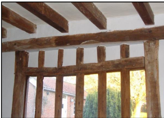
Fig.33 Existing window in hall
