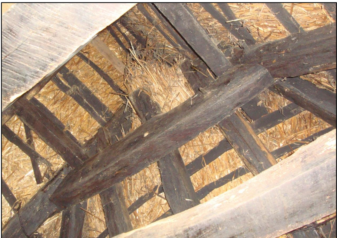
Fig.27 Original vertical gablet at north end of roof
