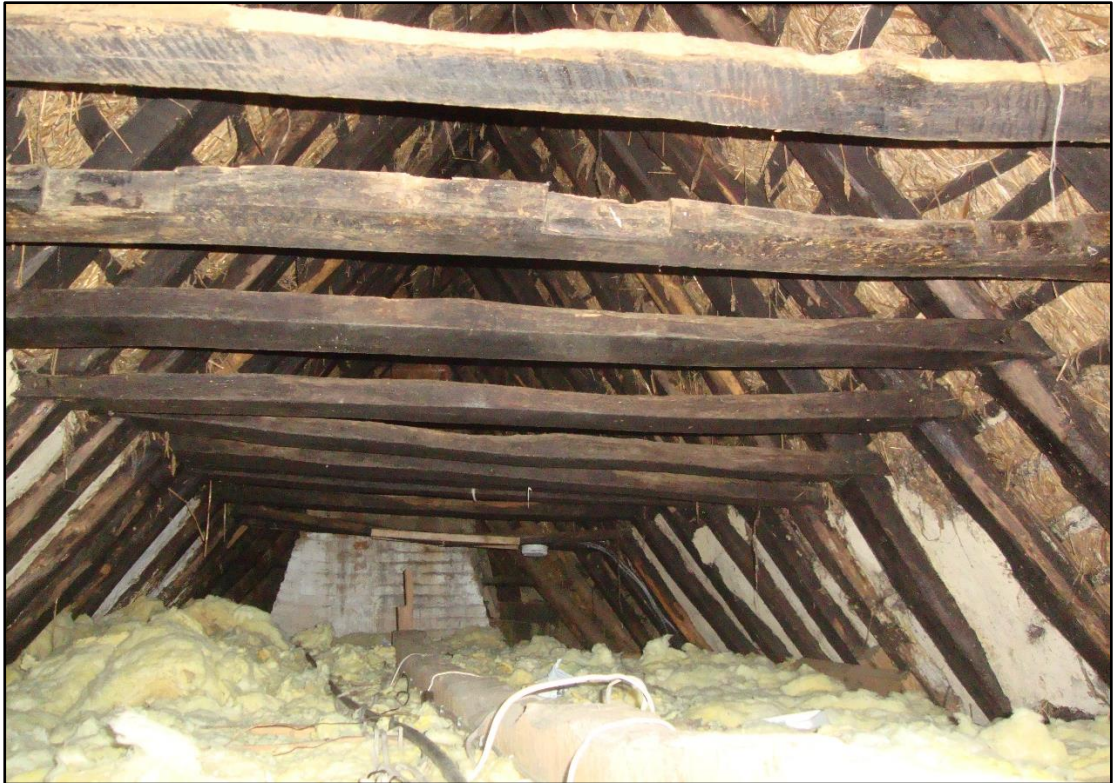
Fig.26 Smoke-blackened components of original collar-rafter roof
