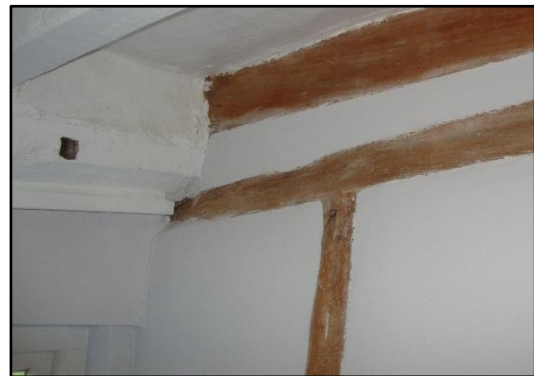
Fig.34 Existing partition in hall
