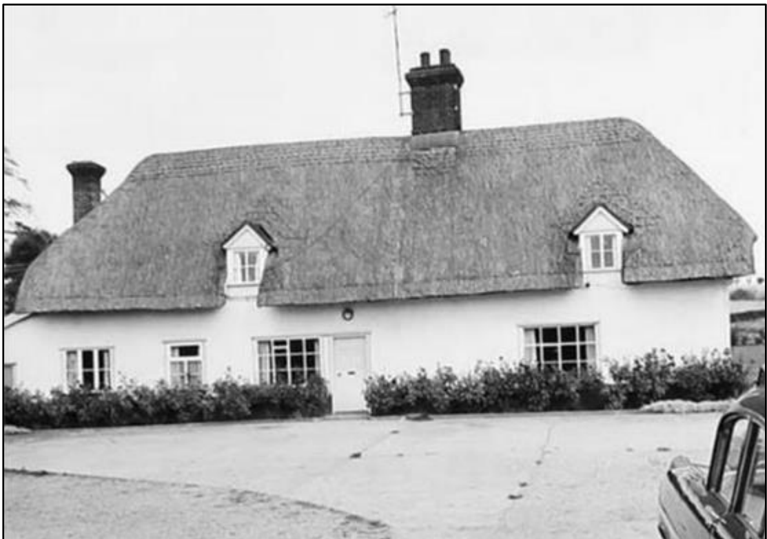
Fig.19 Bridge Farmhouse (NBR 1966)
