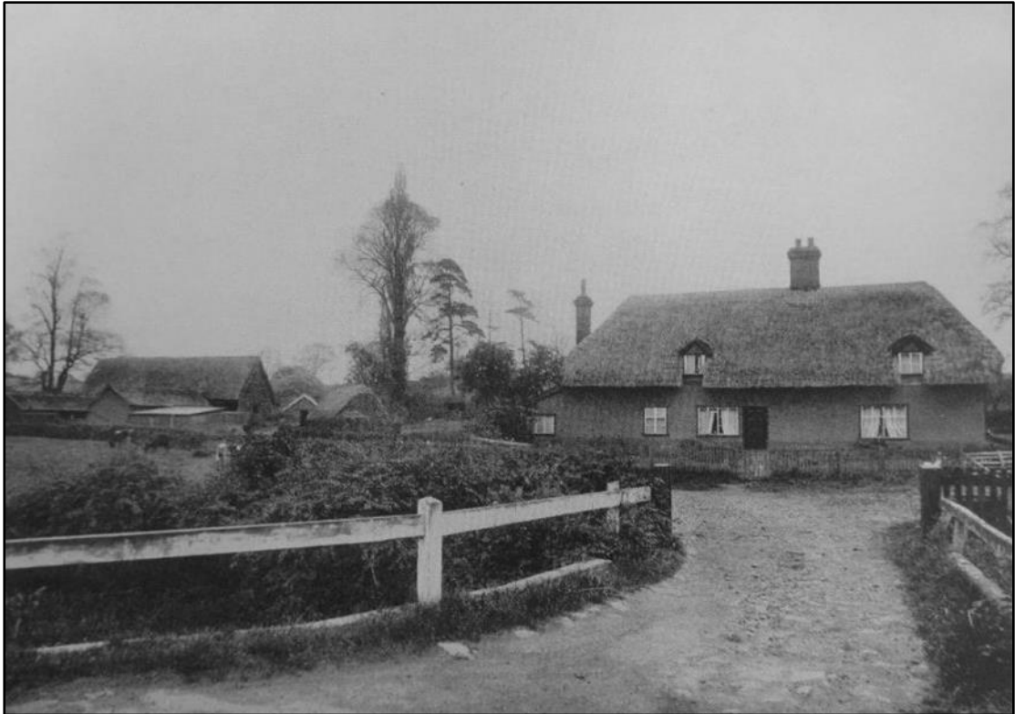
Fig.16 Bridge Farm (c.1936)
