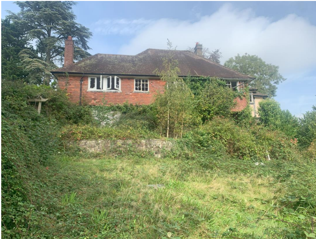
Photograph 1: Rear view of derelict 87 Sidford High Street property showing unkempt rear grassland Area.
