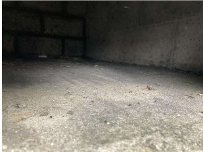
PHOTOGRAPH 17: View of the interior of the coal store
