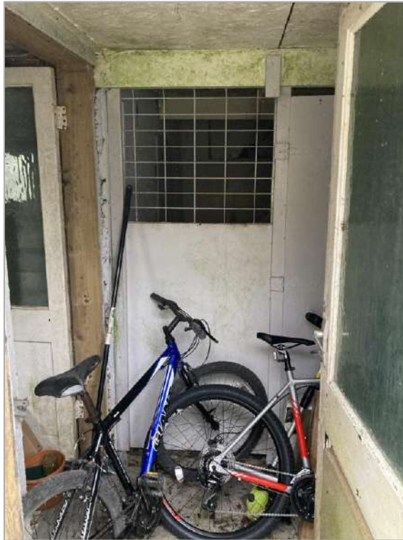
PHOTOGRAPH 11: View of the interior of the outbuilding
