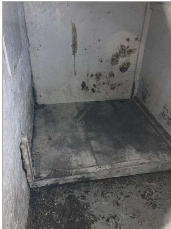
PHOTOGRAPH 13: View of the interior of the outbuilding
