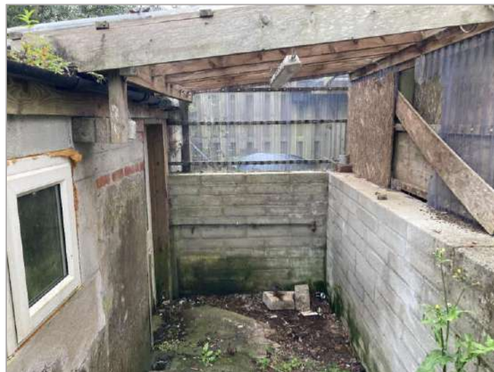
PHOTOGRAPH 10: View of the access to the outbuilding
