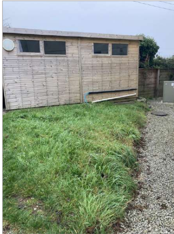
PHOTOGRAPH 15: View of a shed located on the south-eastern boundary of the site
