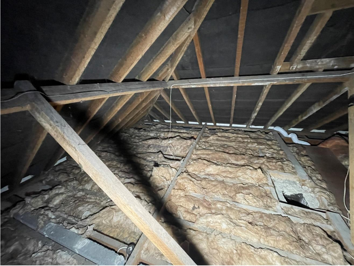
Figure 1 Existing Loft space
