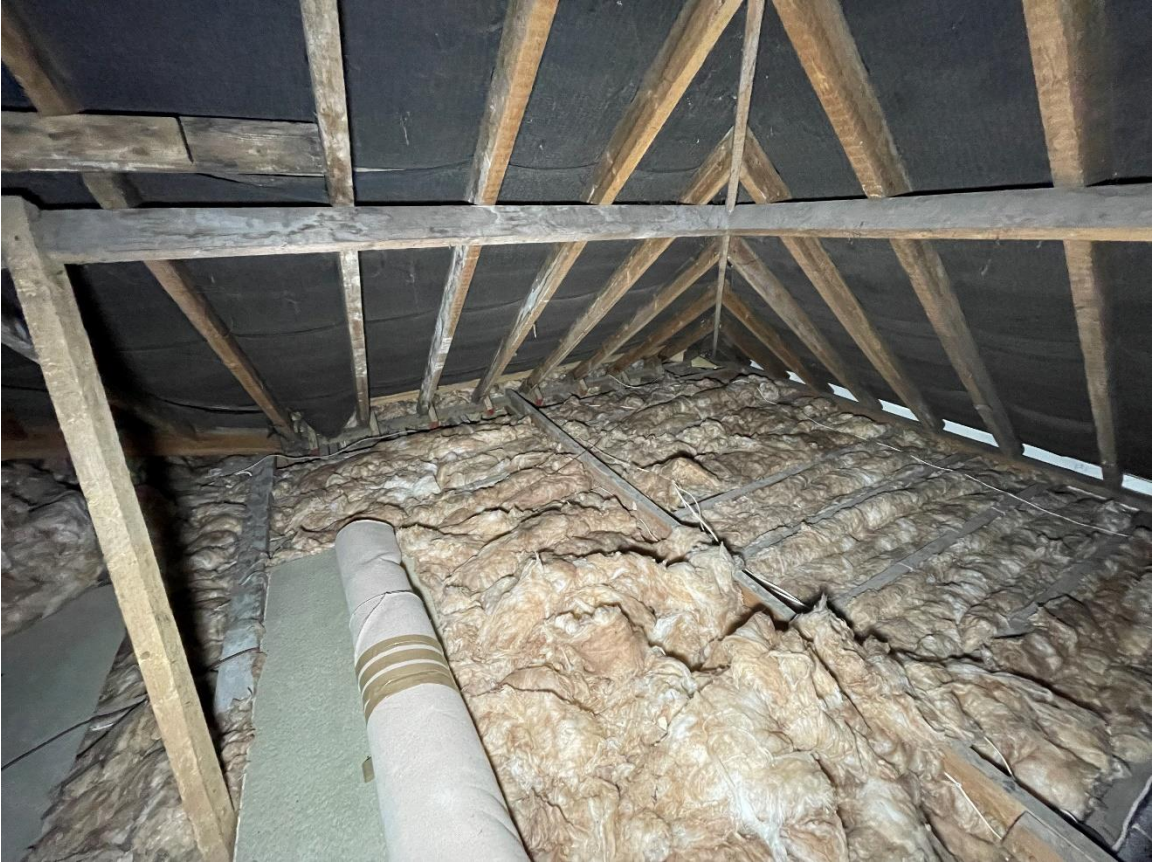
Figure 3 Existing Loft Space
