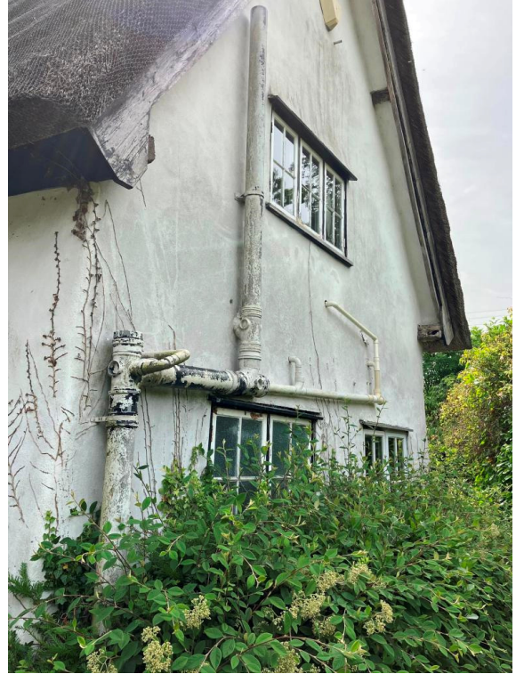
Existing west gable
