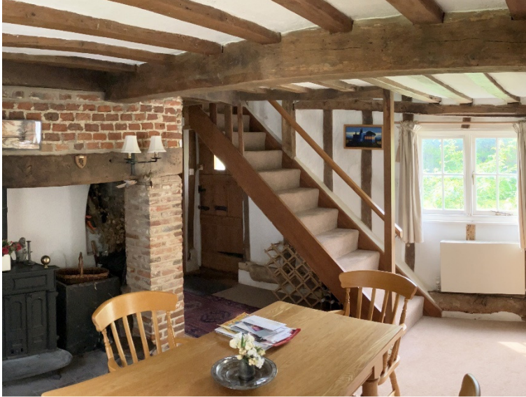
Existing modern stair
