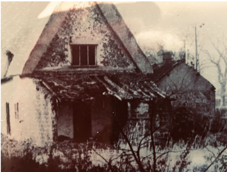
Historic view of east gable, showing former gable window (East lean-to removed previously)
