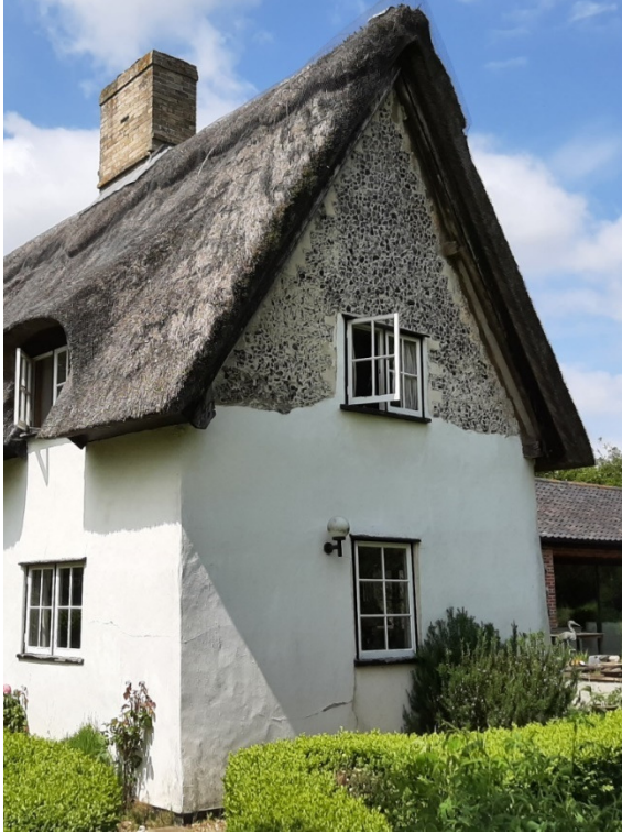
Existing east gable
