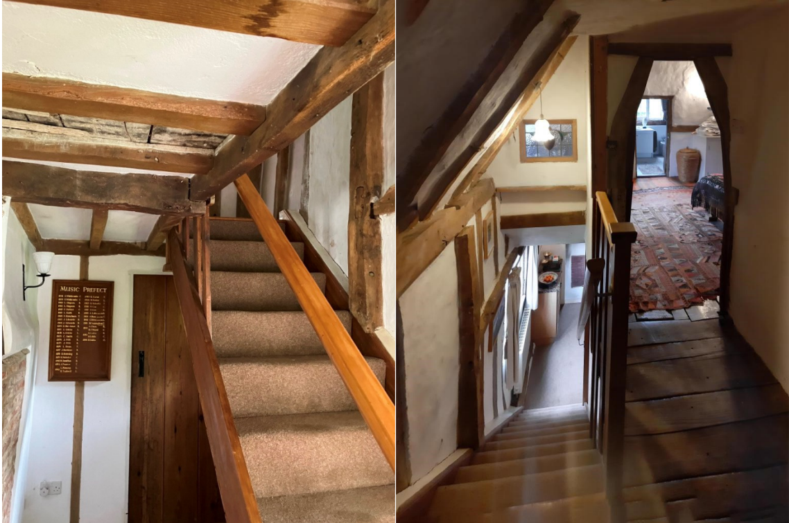
Existing modern stair, showing truncated transverse tie beam.
