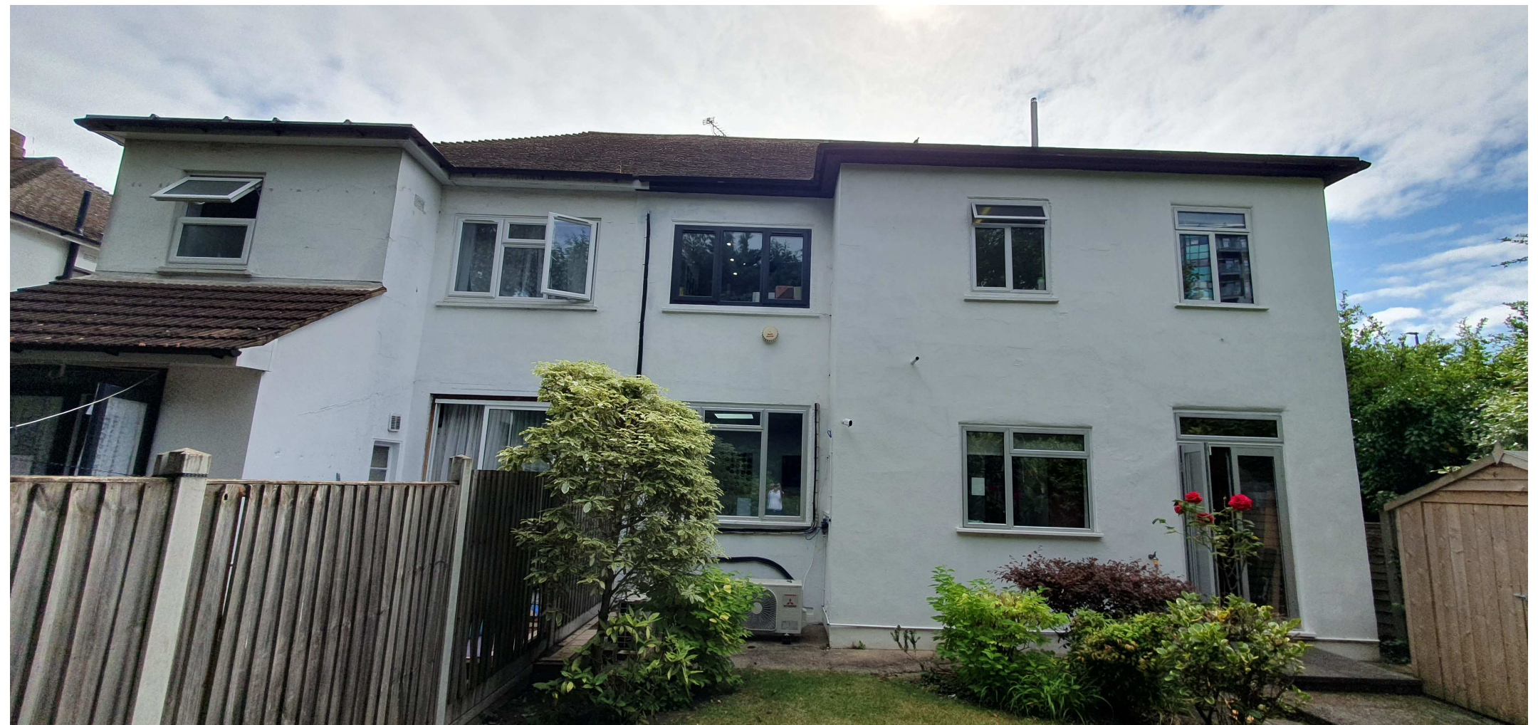
VIEWS OF REAR OF THE PROPERTY
