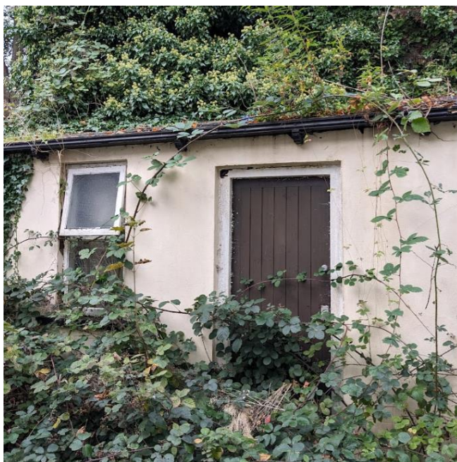
Figure 11 – East elevation of lean-to
