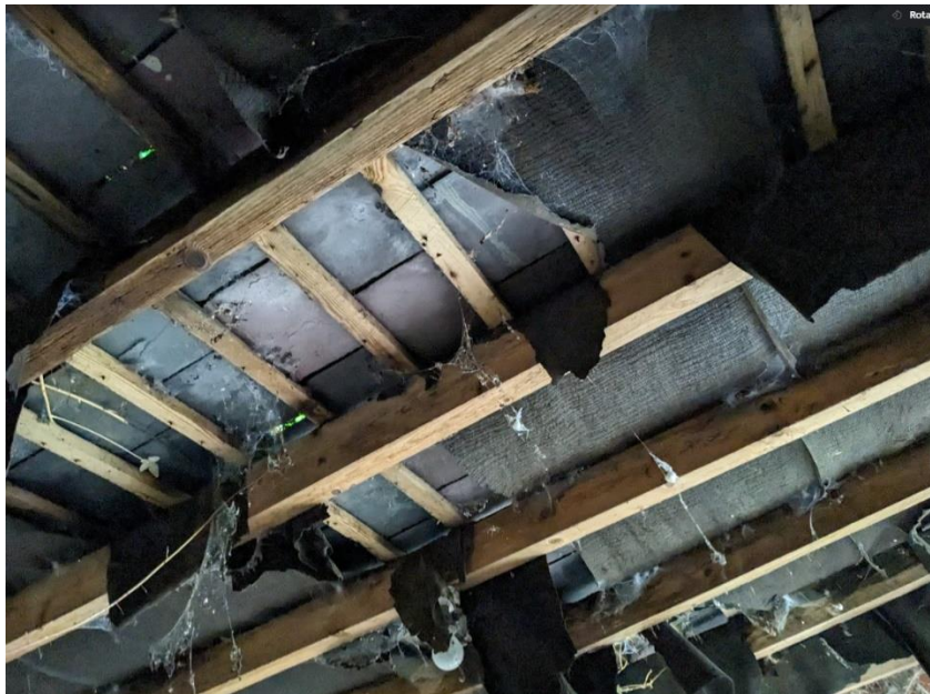
Figure 7 - Underside of east lean-to roof
