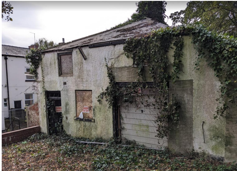
Figure 6 - View of the roof from the north
