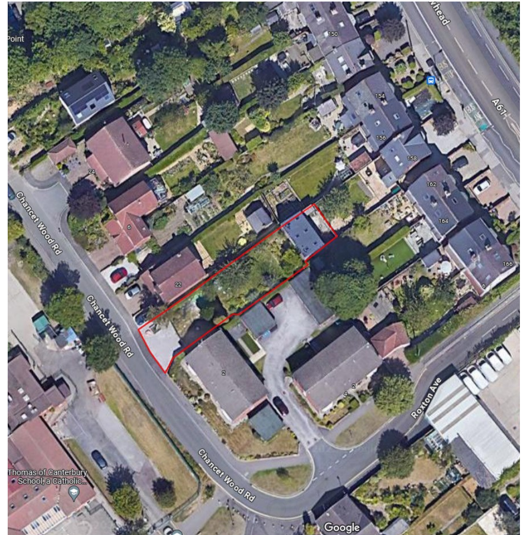
Site location overview
