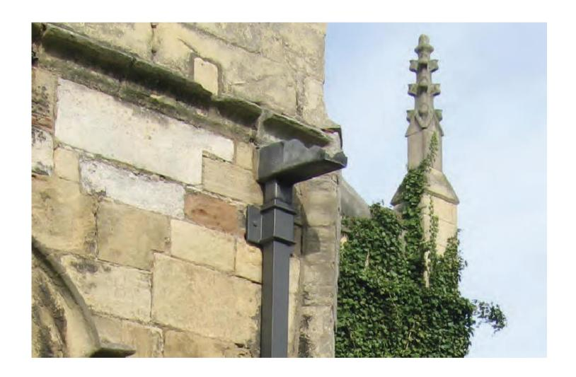
Conduit House, Cowdray Park – Proposal for New Downpipes Below Existing Lead Rainwater Chutes – Indicative Photographic Detail
