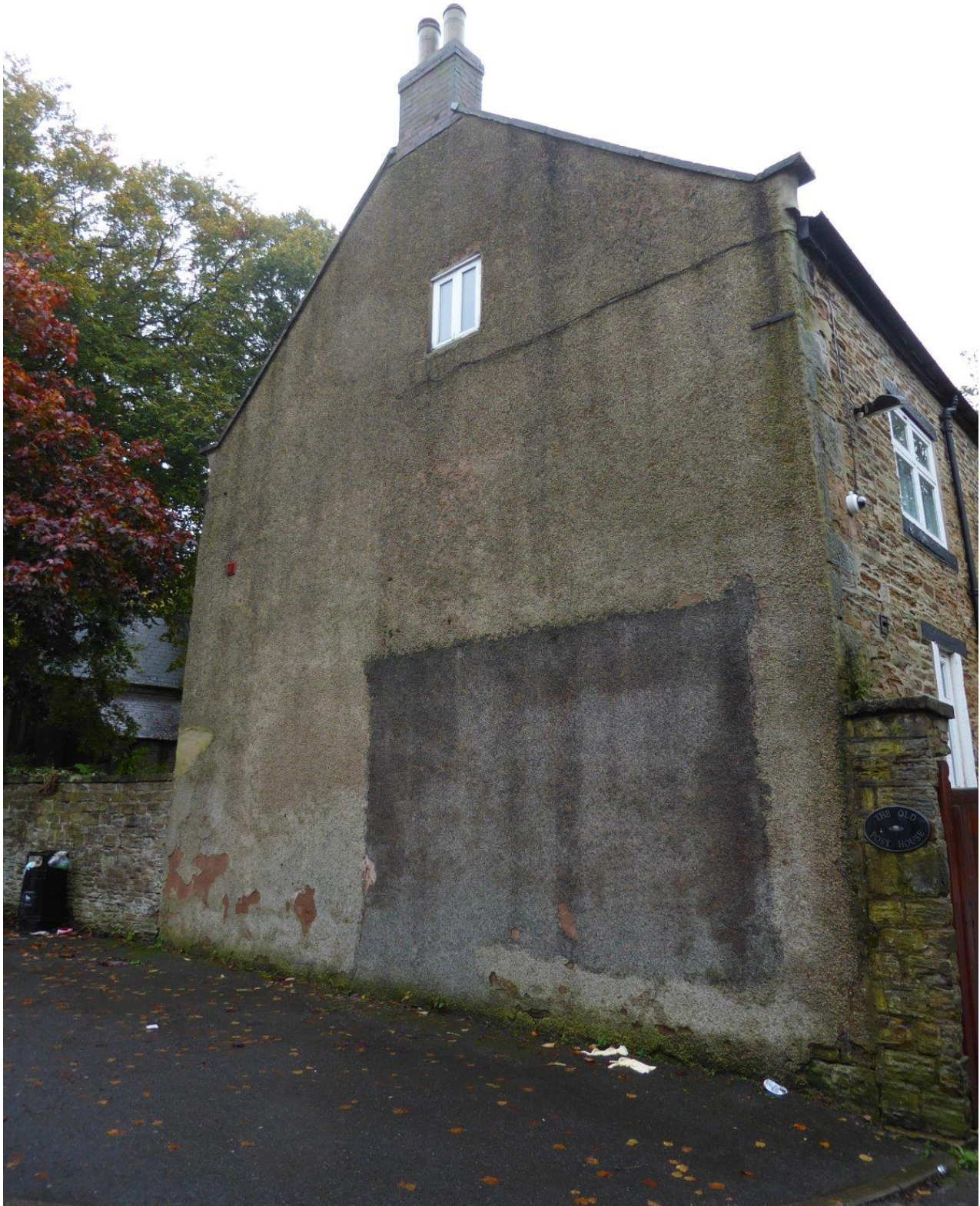
EAST GABLE END
