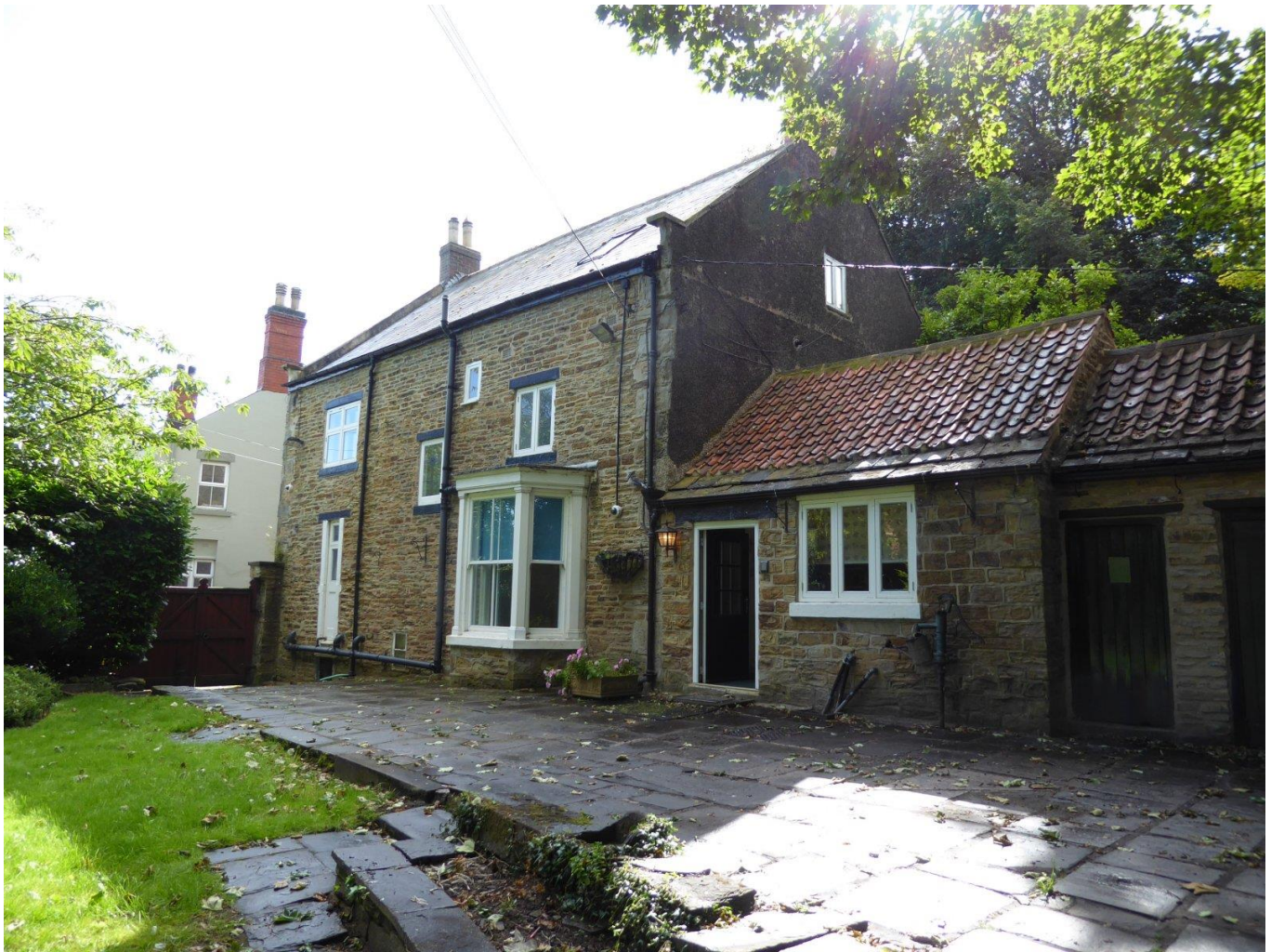
REAR (NORTH) SIDE SHOWING WEST GABLE
