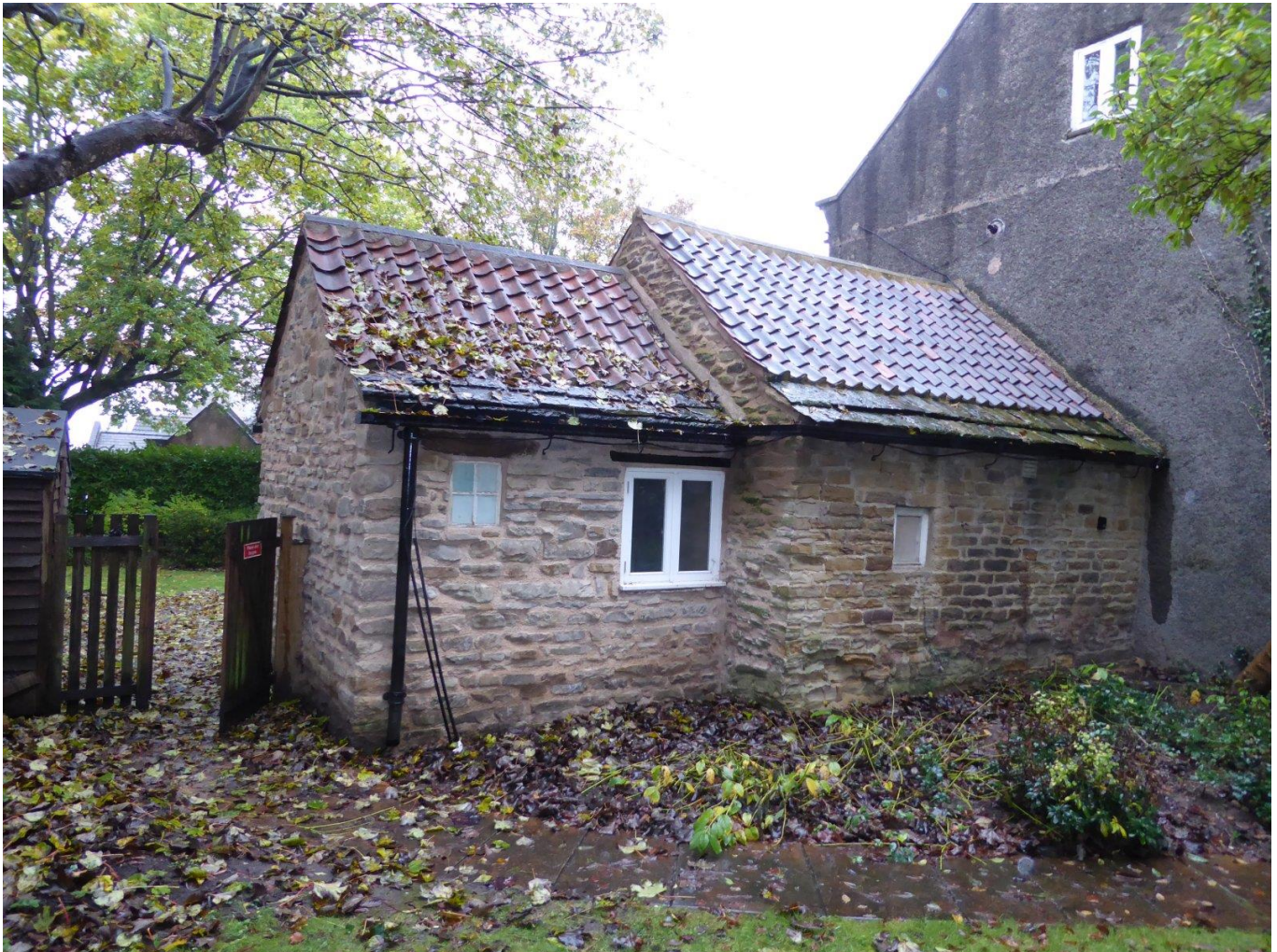
EXISTING EXTENSIONS, SOUTH SIDE
