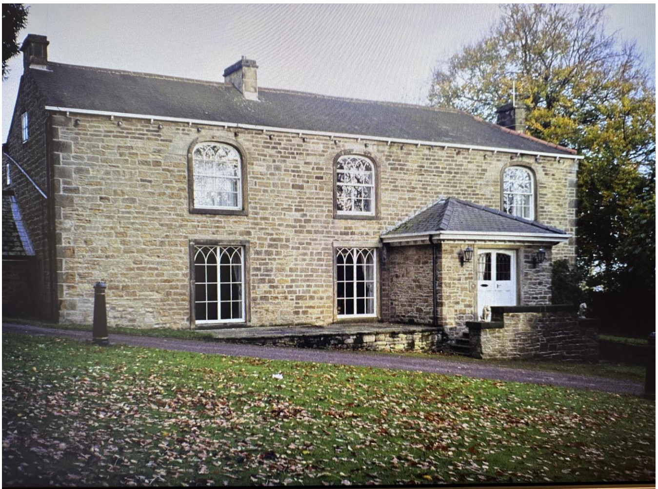
ELMWOOD HOUSE, HOLLINGWOOD, CHESTERFIELD
