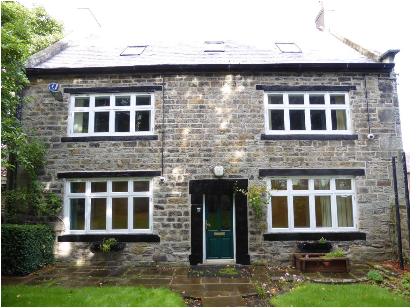
FRONT (SOUTH) SIDE
