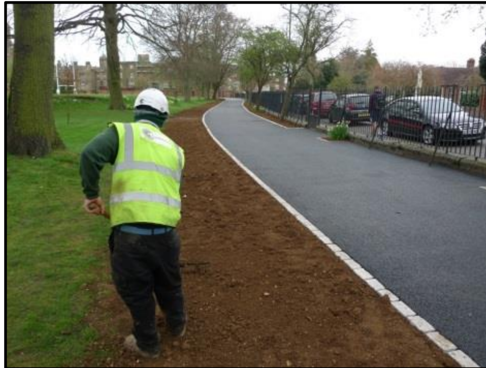
Fig 15 – All 'making good' topsoil will be BS3882 compliant and raked out by hand to no greater depth than 100mm.
