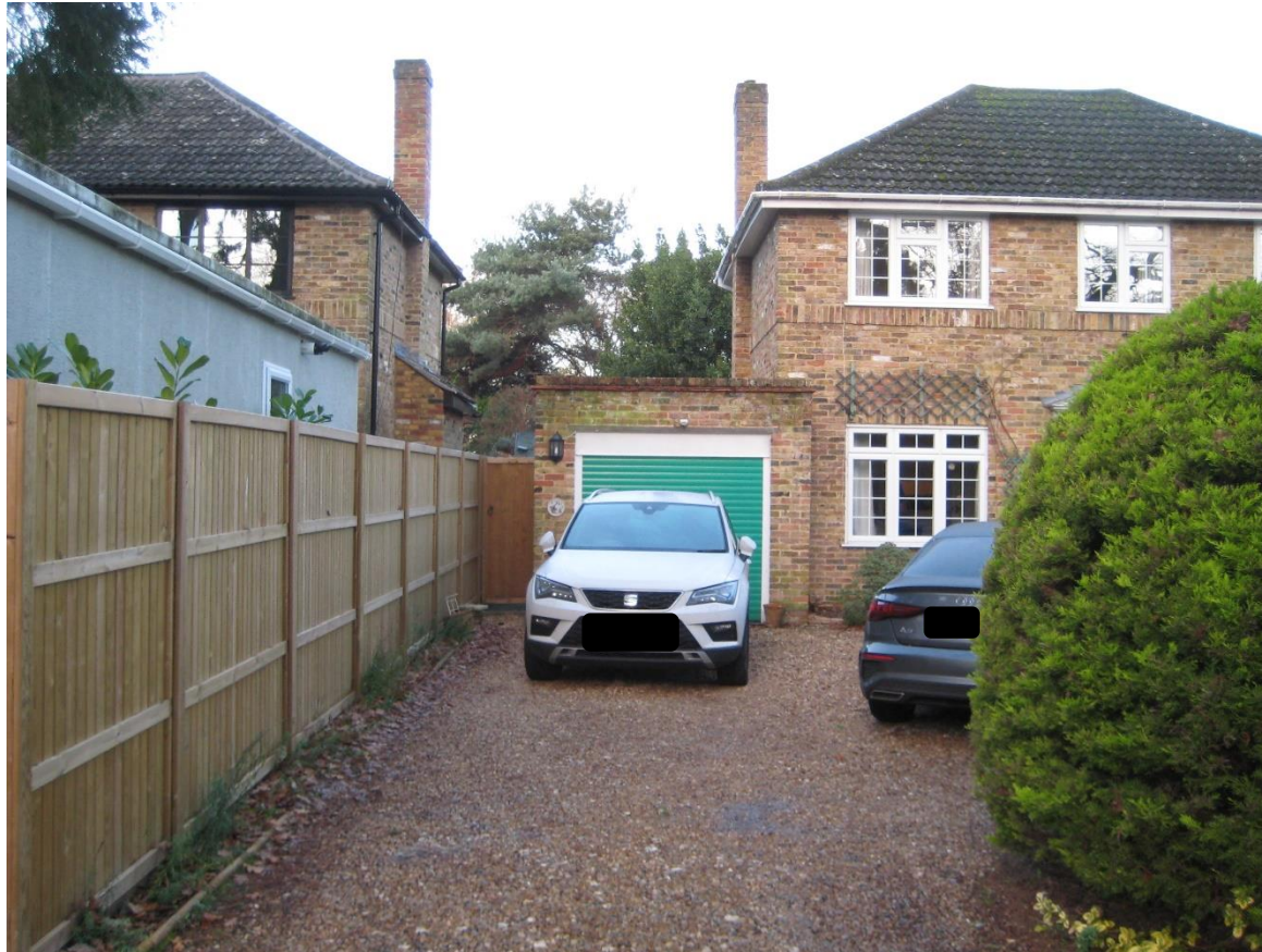
Fig 10 – Existing front driveway area. Temporary ground protection will supplement this given likely parking/ site storage. Note: Garage to be demolished is visible.
