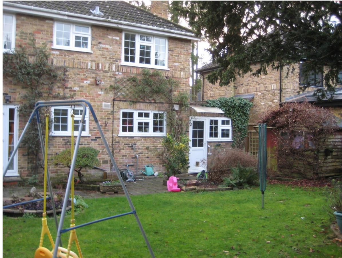
Image 1 – Looking towards area of side extension from rear garden.
