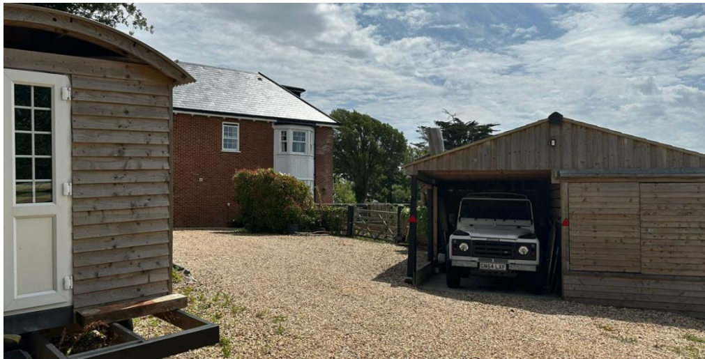
Image 4 – Photograph showing an existing garage/car port to be demolished to accommodate the proposed dwelling.
