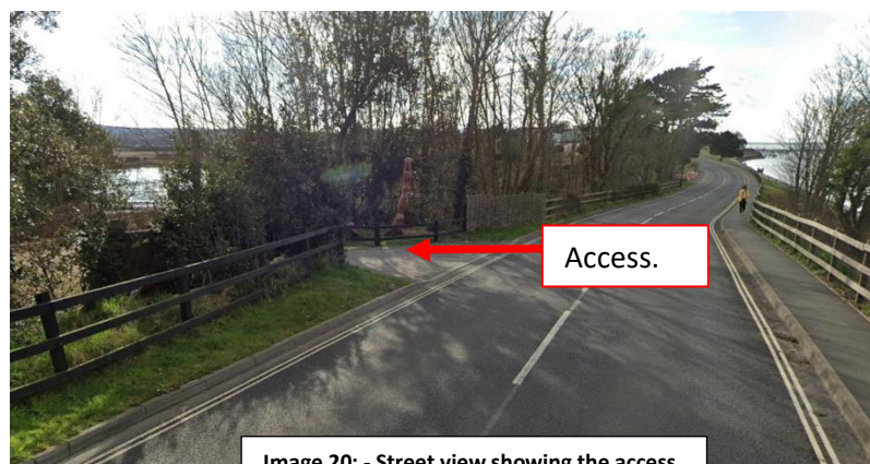
Image 20: - Street view showing the access.
