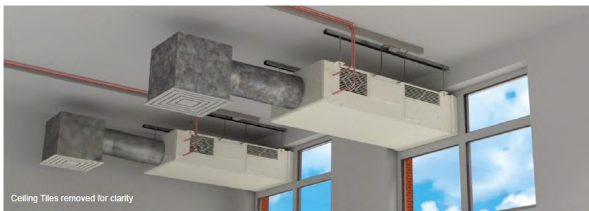
FIGURE 9: EXAMPLE OF HYBRID VENTILATION UNITS
