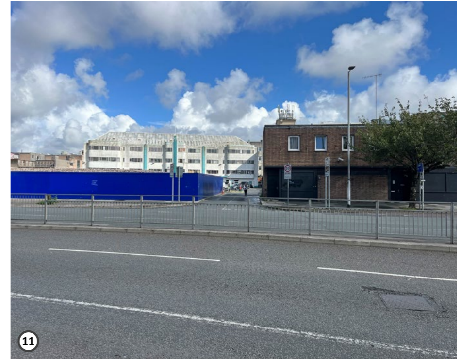
View towards CCC access road from Western Approach
