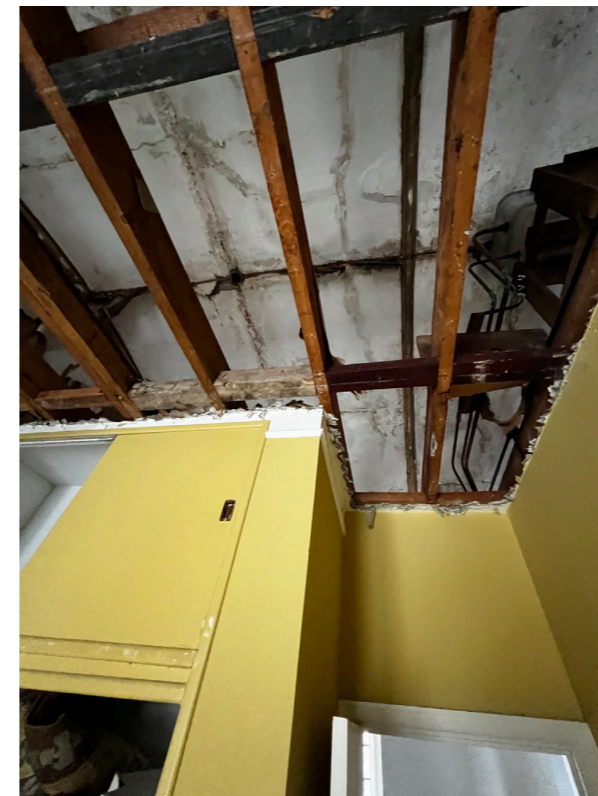
Existing concrete ceiling
