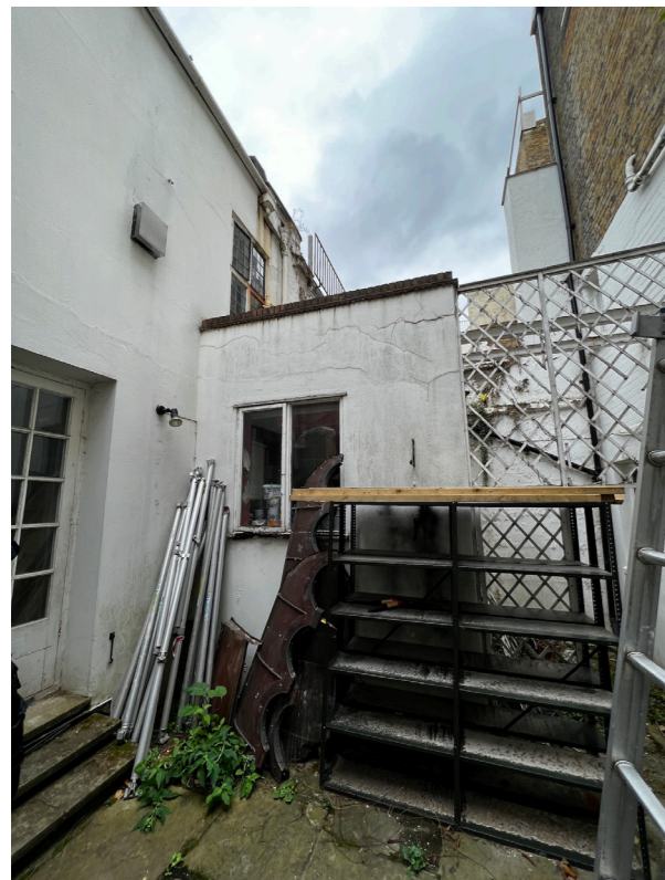
Existing rear single-storey extension
