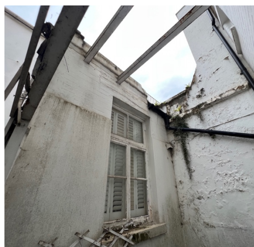
Rear extension and garden boundary wall
