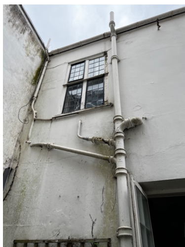
Current condition of the existing building
