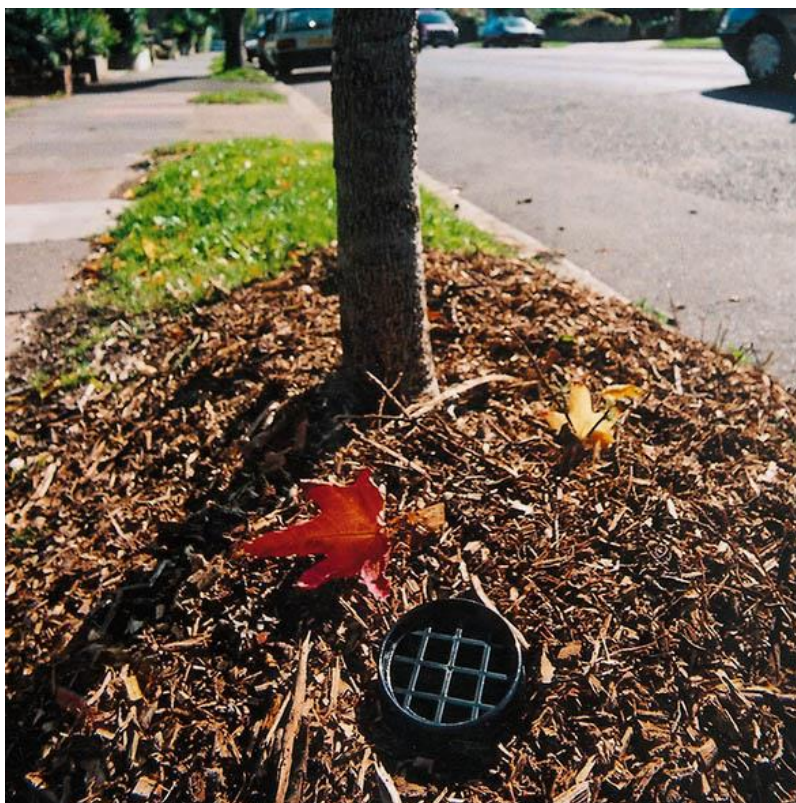
Photo 2: Example of a tree with an irrigation system installed. The grid lid is present at ground level. Copyright to Green Blue Urban (2021)
