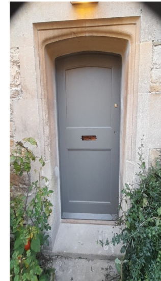
New door to match existing door to Number 5
