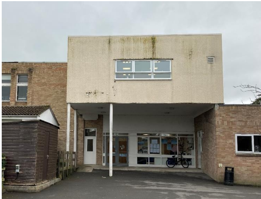
Existing Extension to be re clad new composite deck and balustrade below
