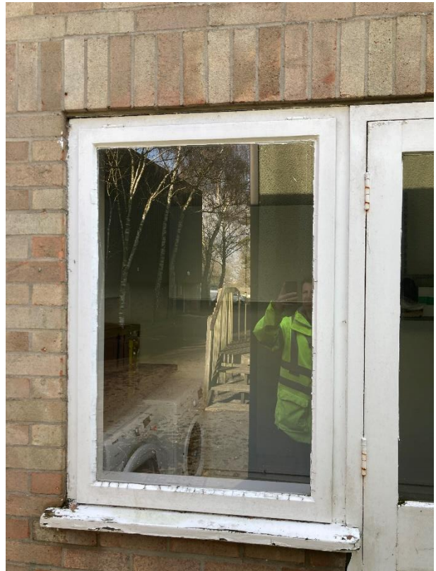
Typical condition of Existing Windows
