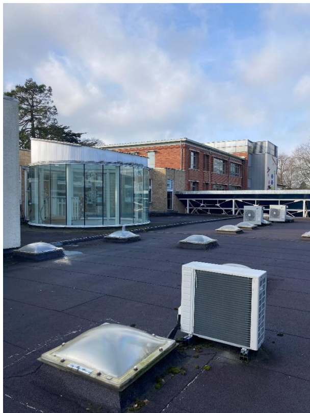
Existing Flat roofs
