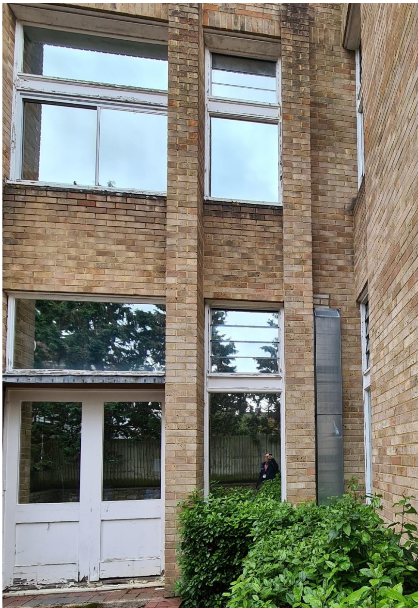
Typical existing windows and doors to be replaced
