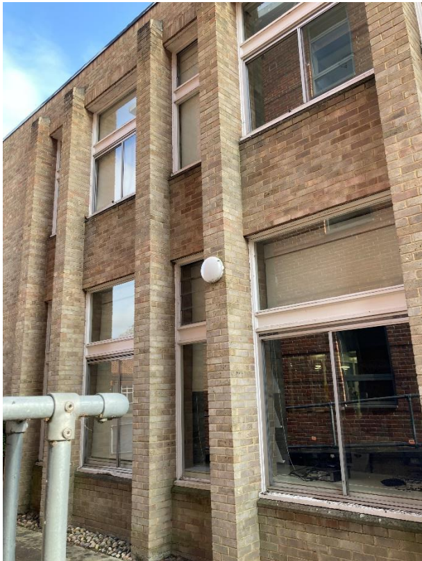
Typical facing brick façade and Windows
