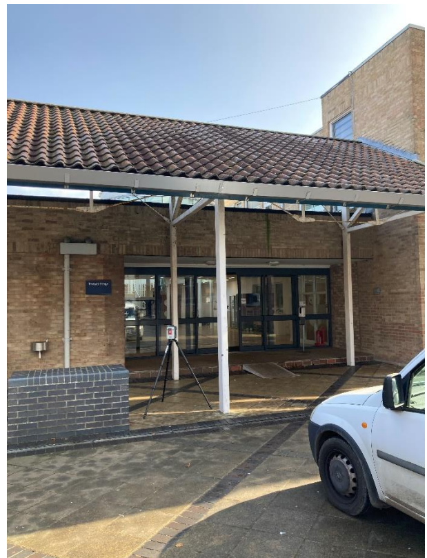
Main Entrance – no works proposed
